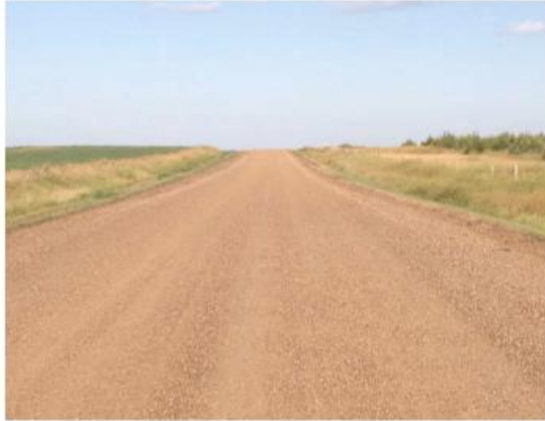
Figure 3.20 Gravel road with adequate crown
