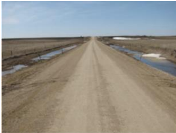
Figure 3.22 Gravel road with excessive crown
