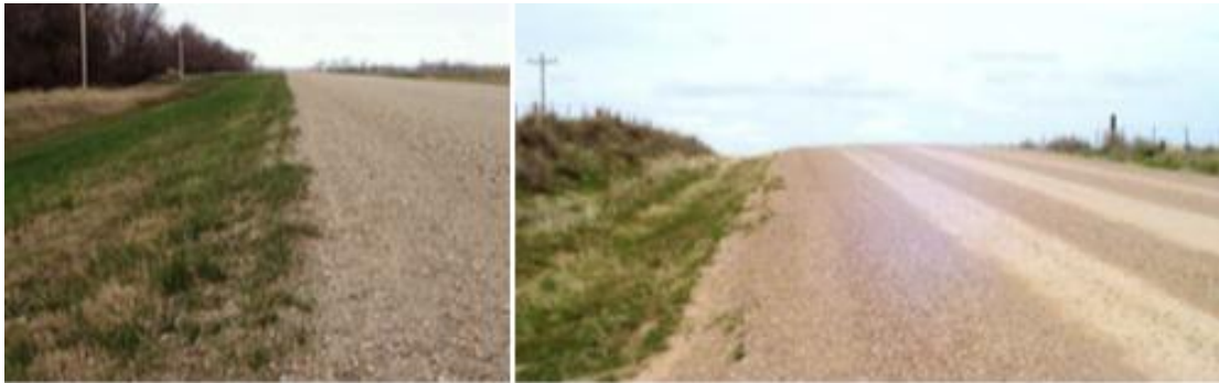
Figure 3.23 Gravel road with good condition shoulders
