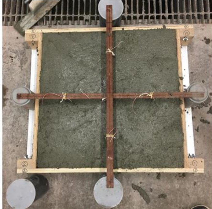
Figure 3.5 Casting of bulk concrete panel and placement of embedded PZT cement modules
