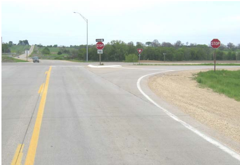
Figure 1: Illustration of how an island can be used to place an additional stop sign at an intersection.
