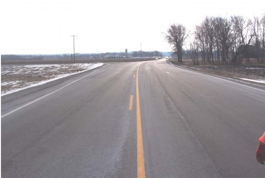
Figure A1: A view of Cox Road intersection facing east on the Whitewater Bypass.
