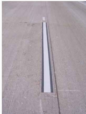
Figure 4: Two types of pavement markings used together on the Oconomowoc Bypass illustrate a very visible treatment in various situations.
