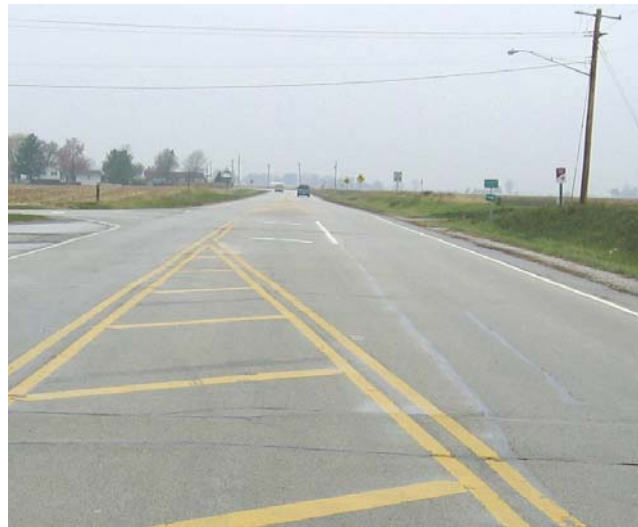
Figure 2: Typical example of a marked left turn lane on a 2-lane roadway.
