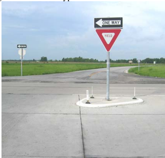
Figure 7: Second crossing right of way control at in a median in Missouri.
