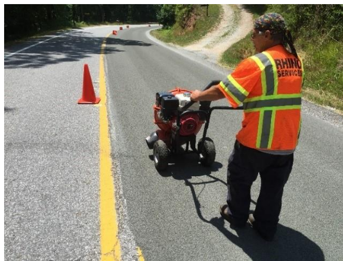
Figure 7 – Picture. Excess aggregate removal with mechanical blower.
