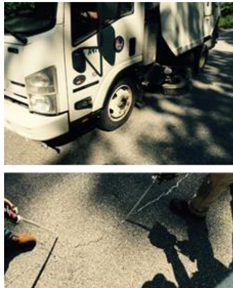
Figure 4 – Pictures. Surface cleaning (top) and cracks sealing with epoxy (bottom).
