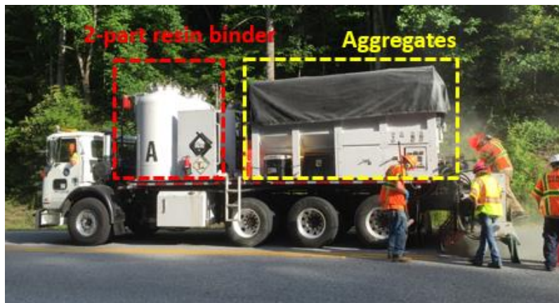
Figure 5 – Picture. Designated truck in operation, automatically placing HFST binder and aggregates.
