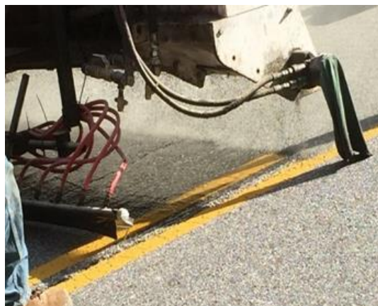
Figure 6 – Picture. Close up of automatic binder and aggregates placement.
