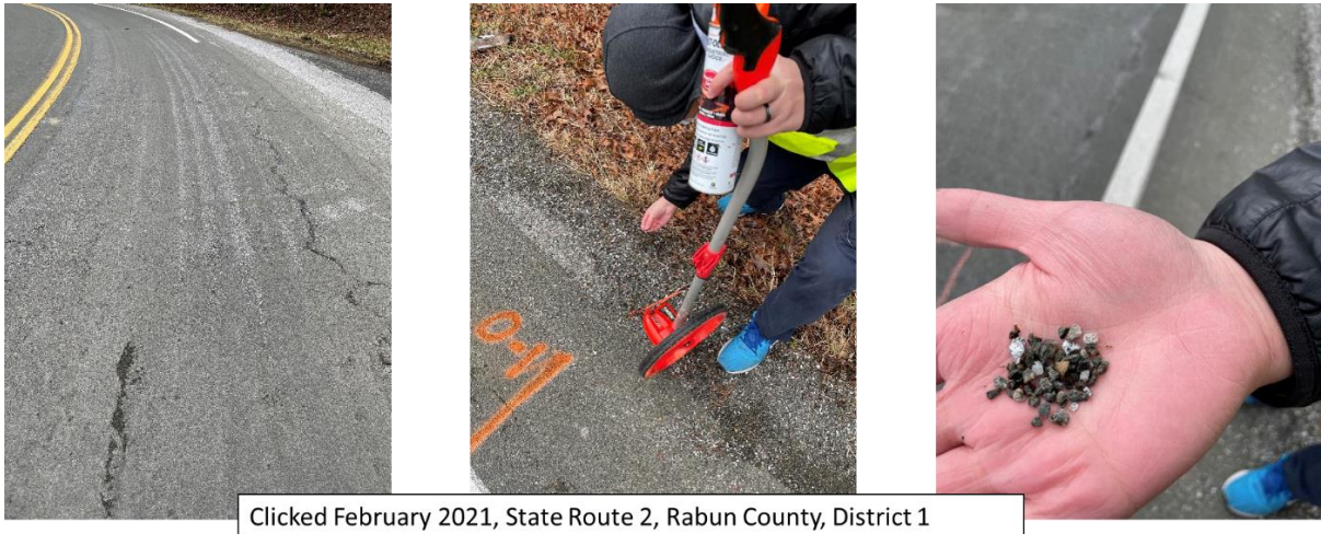
Figure 57 – Pictures. Aggregate loss on the wheel path as well as dislodged aggregates on the shoulder.
