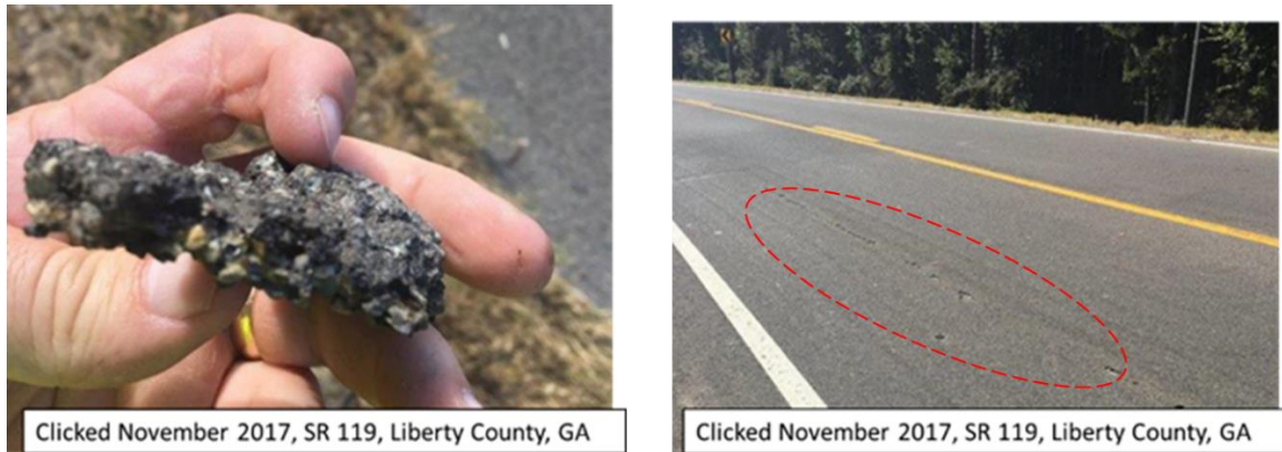
Figure 54 – Pictures. Asphalt pavement pop-off along with HFST layer in SR 119, Liberty County, GA. (this site has been replaced).
