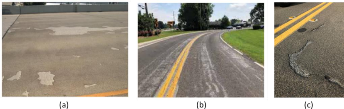
Figure 10 – Pictures. Examples of different HFST distresses: (a) HFST delamination (FDOT, 2019), (b) HFST aggregate loss (Courtesy of KYTC), and (c) Pavement pop-off with attached HFST (photographed by author).
