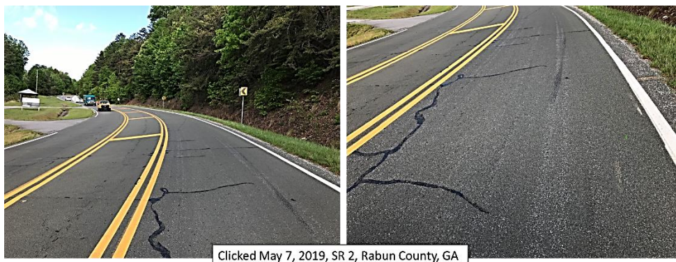
Figure 57 – Pictures. Aggregate loss on the wheel path as well as dislodged aggregates on the shoulder.
