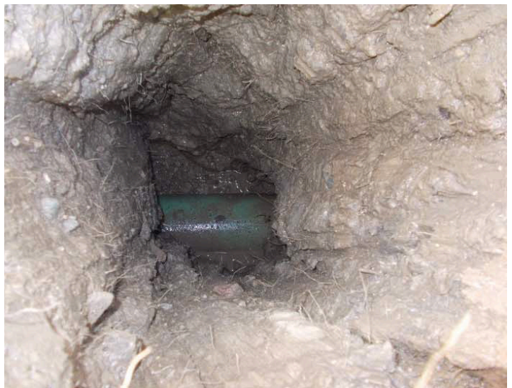
Figure 6. Gas Main exposed through Vacuum Excavation.
