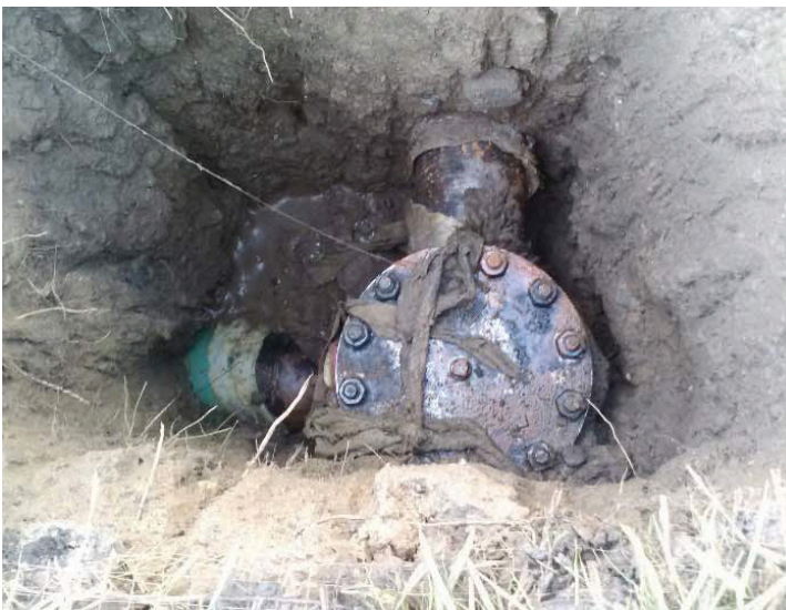
Figure 6. Gas Main exposed through Vacuum Excavation.
