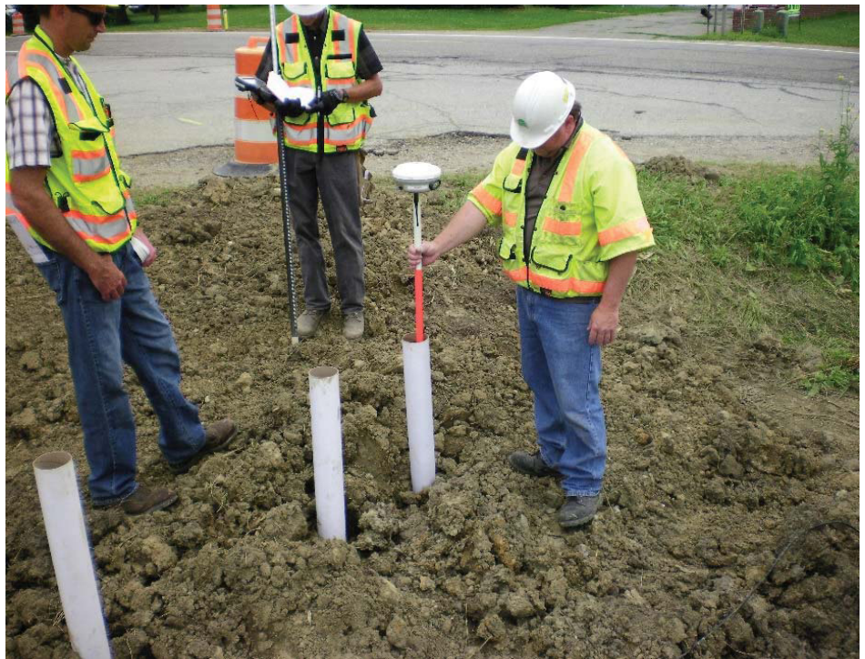
Figure 5. Michigan DOT utility crew surveying inside cardboard tubes after backfill.
