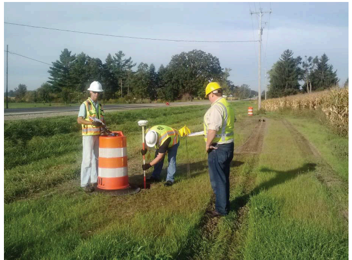
Figure 6. Survey crew obtaining positional data on exposed utility.
