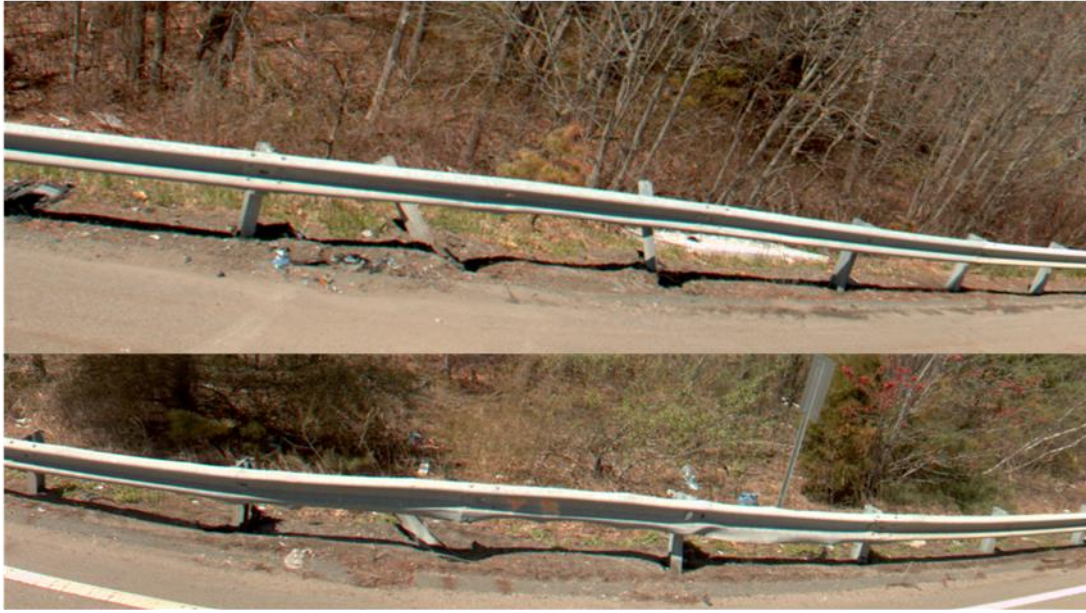
Figure 3.5: Examples of identified support failures
