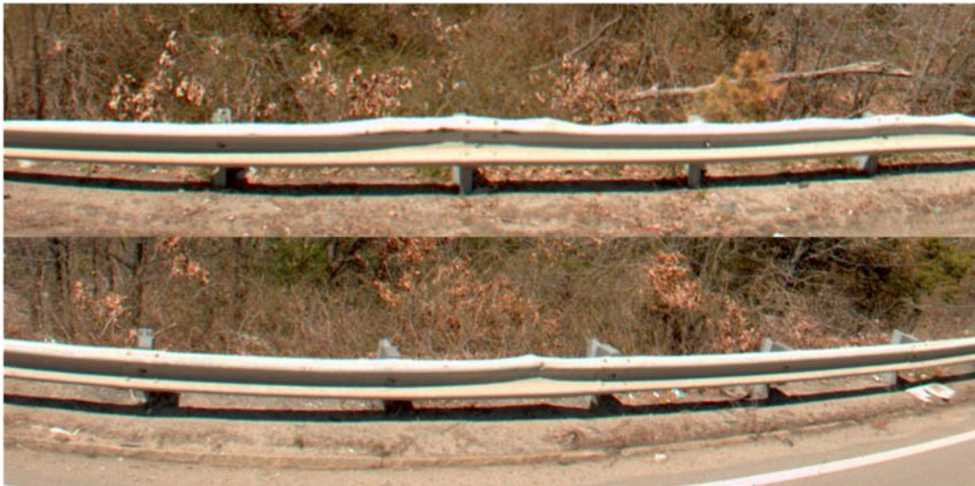
Figure 3.4: Examples of the identified face dentations
