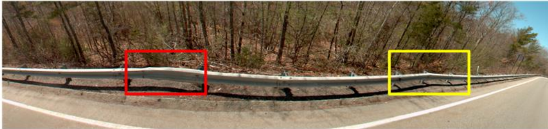
Figure 2.18: Identified sections with face dentations
