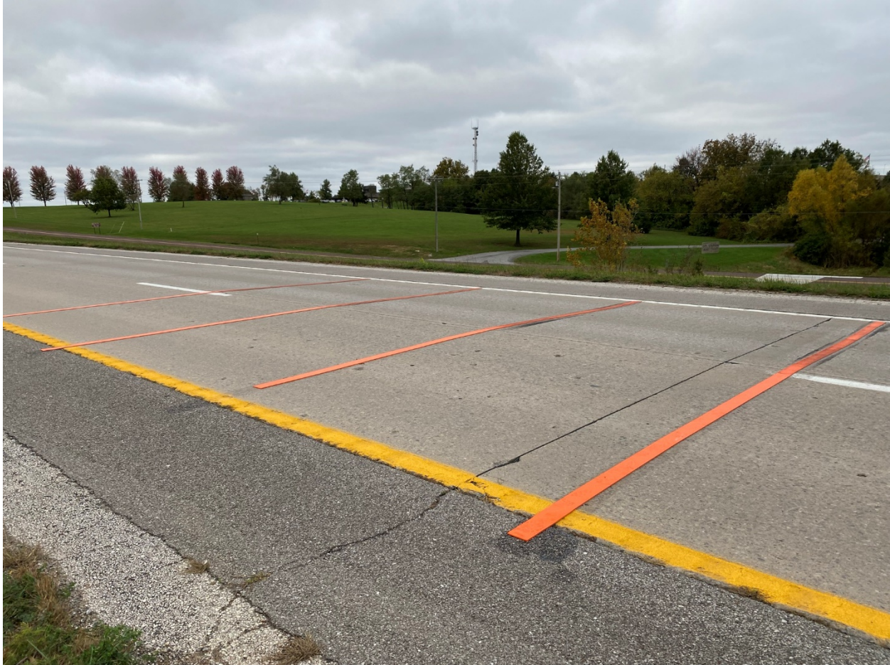
Figure 1-2. Long-term temporary rumble strips installed on US 63 southbound in Columbia
