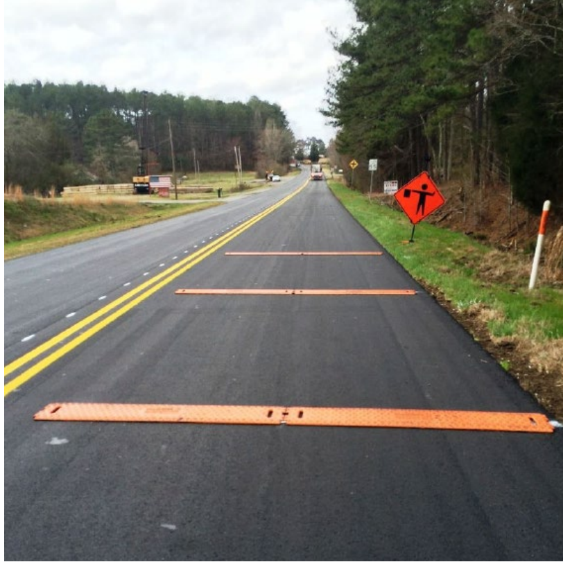
Figure 3-5. Example TPRS layout and flagger signage on State Route (SR) 20 in Floyd County, Georgia
