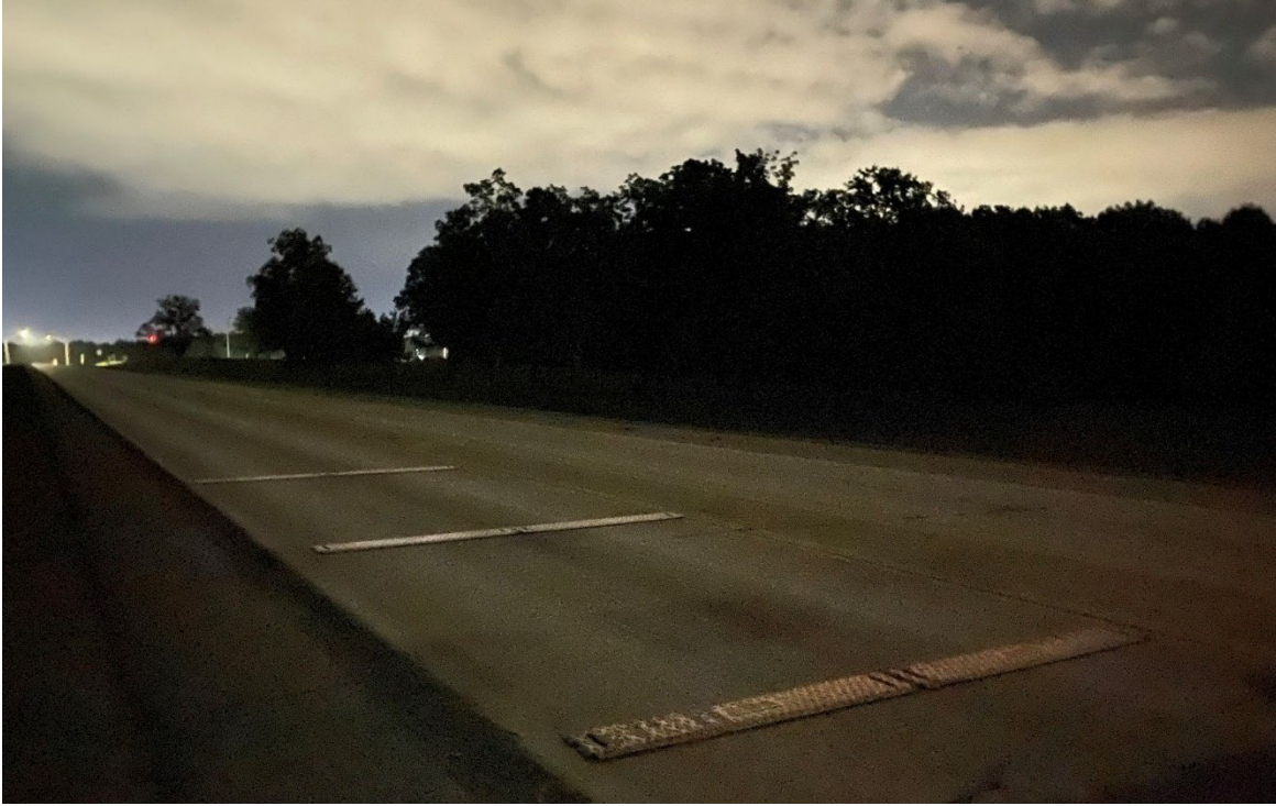
Figure 5-2. Short-term temporary rumble strips on US 24 in Moberly
