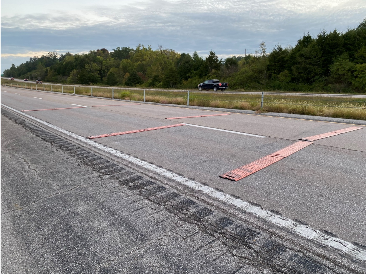
Figure 1-1. Short-term temporary rumble strips installed on US 63 southbound in Ashland
