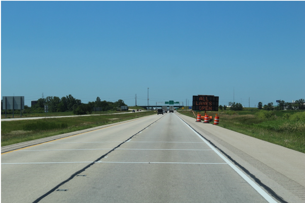
Figure 3-6. Example Illinois Department of Transportation (IDOT) deployment of long-term temporary rumble strips [temporary rumble strips (special)]
