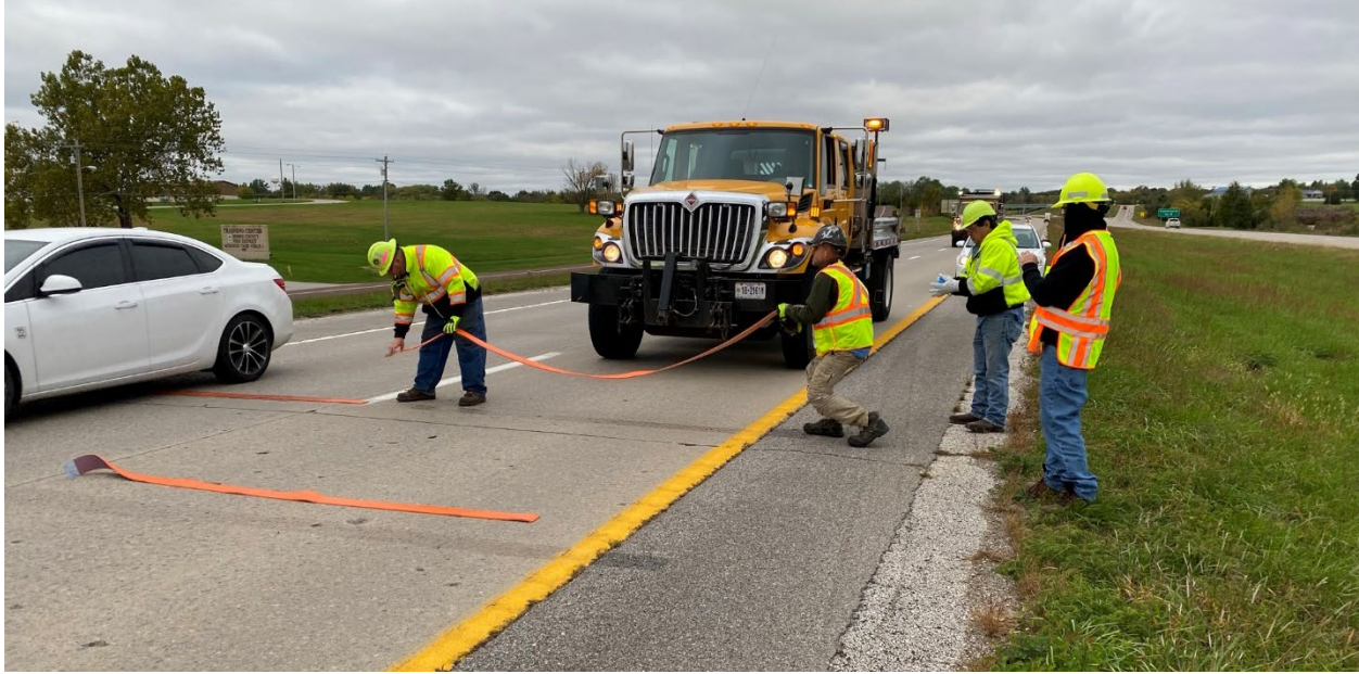
Figure 5-9. Installation of long-term temporary rumble strips on US 63 near Columbia
