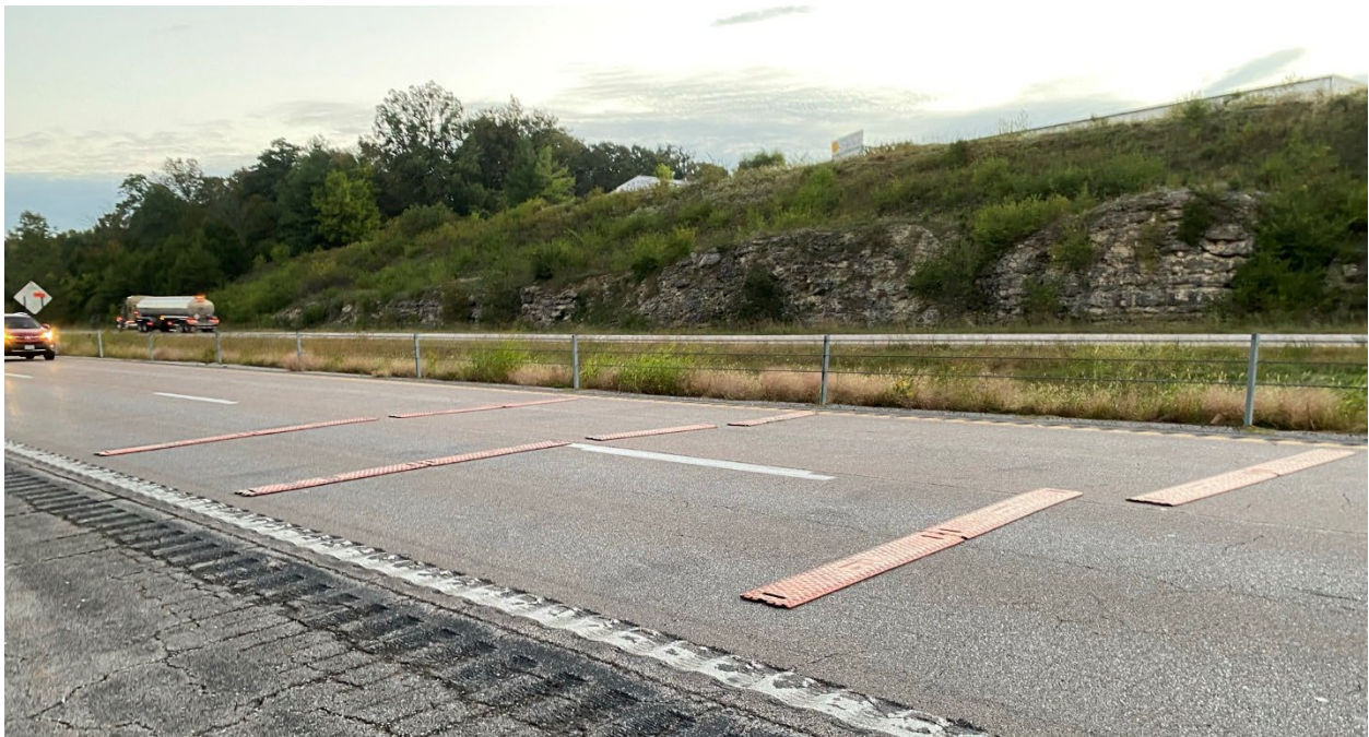
Figure 5-8. Short-term temporary rumble strips on US 63 near Ashland
