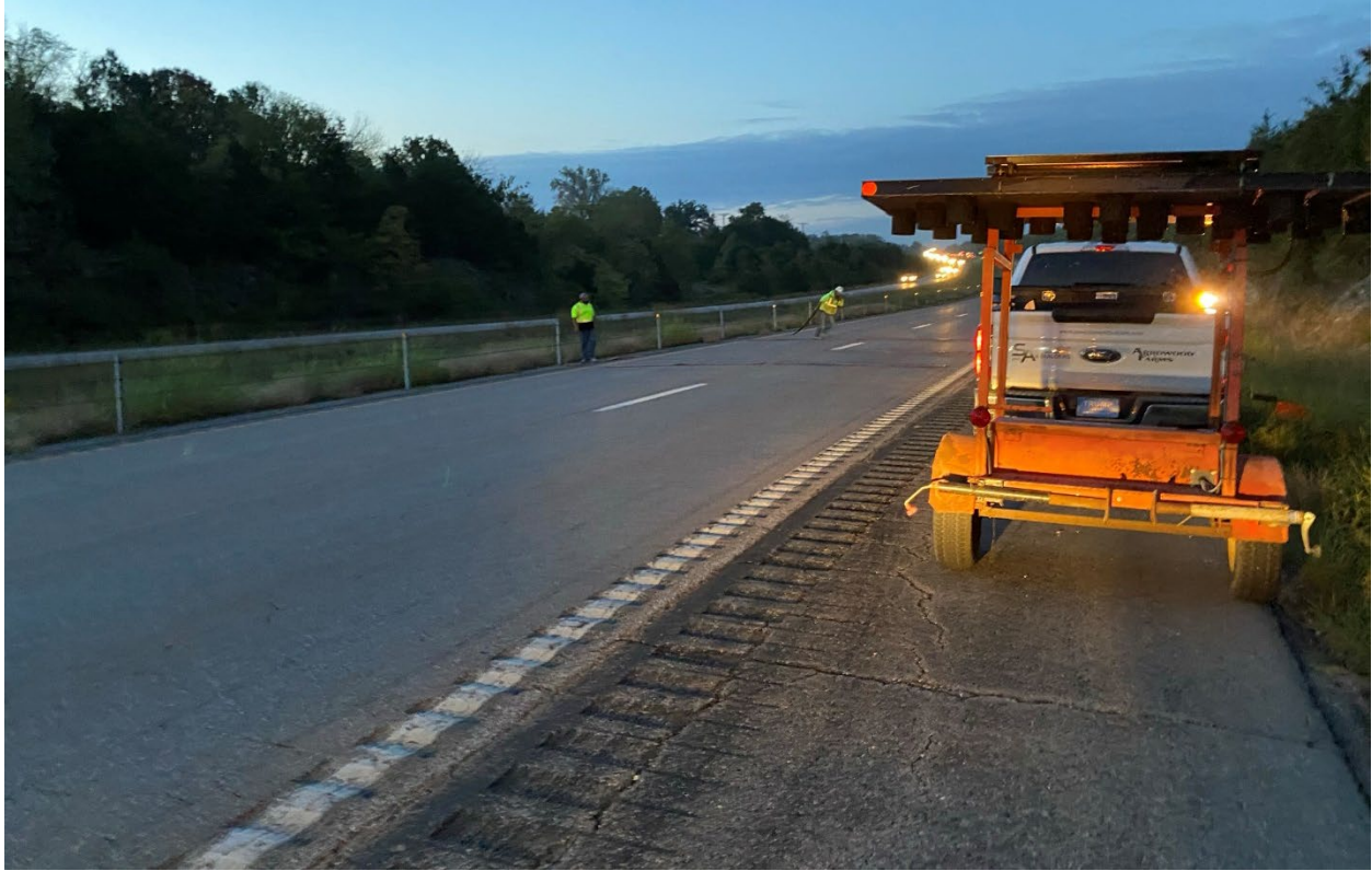
Figure 5-7. Installation of short-term temporary rumble strips on US 63 near Ashland
