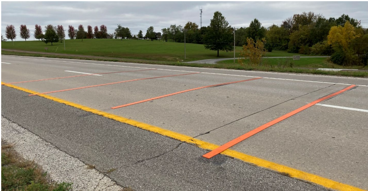
Figure 5-10. Long-term temporary rumble strips on US 63 near Columbia
