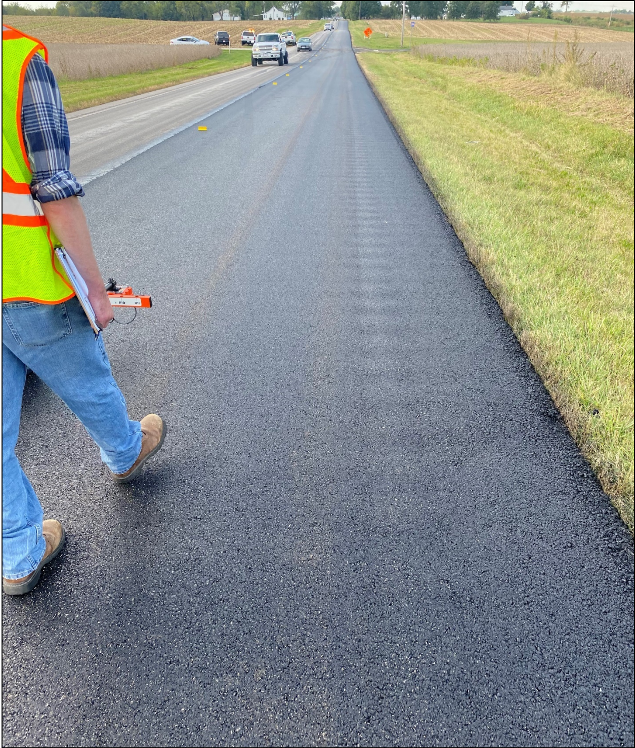
Figure 15. Photo. Rumble strips are shown reflecting through the overlay.
