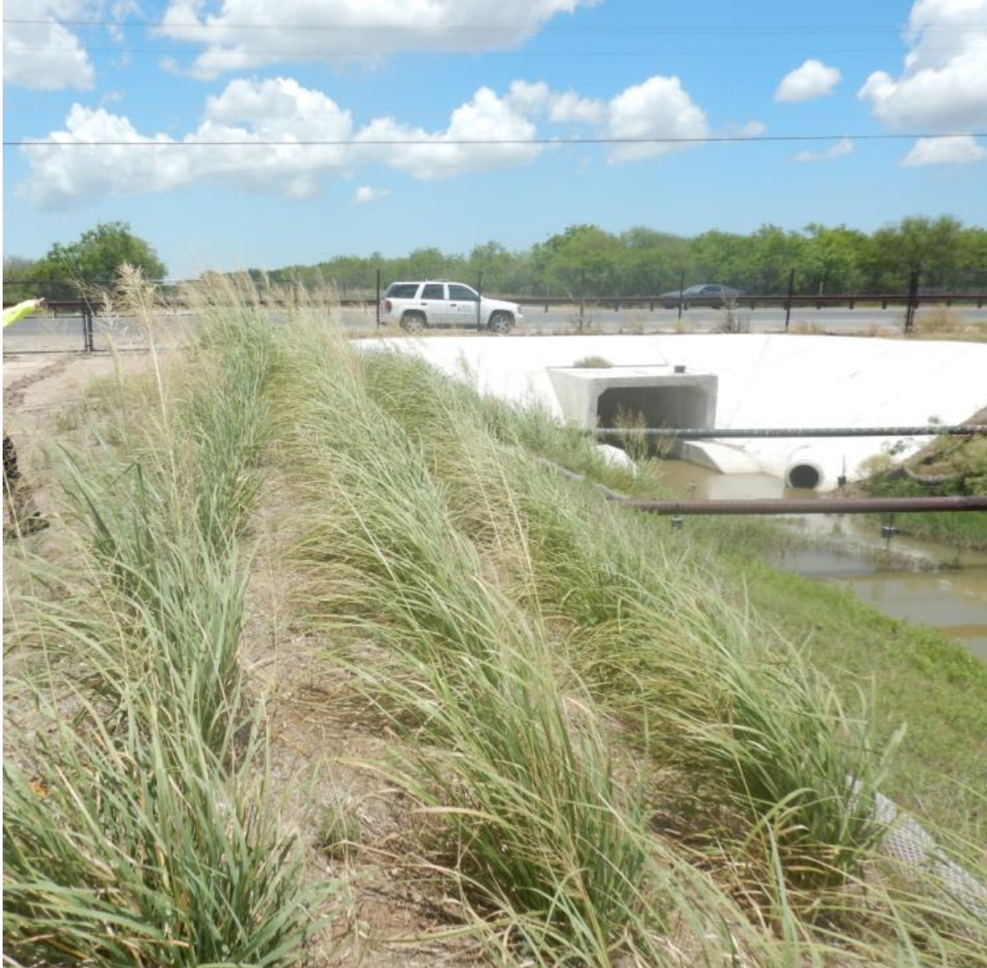
Figure H.16: Wildlife Crossing #2 on SH 100 with Step and Ramp and vegetation planted on the banks
