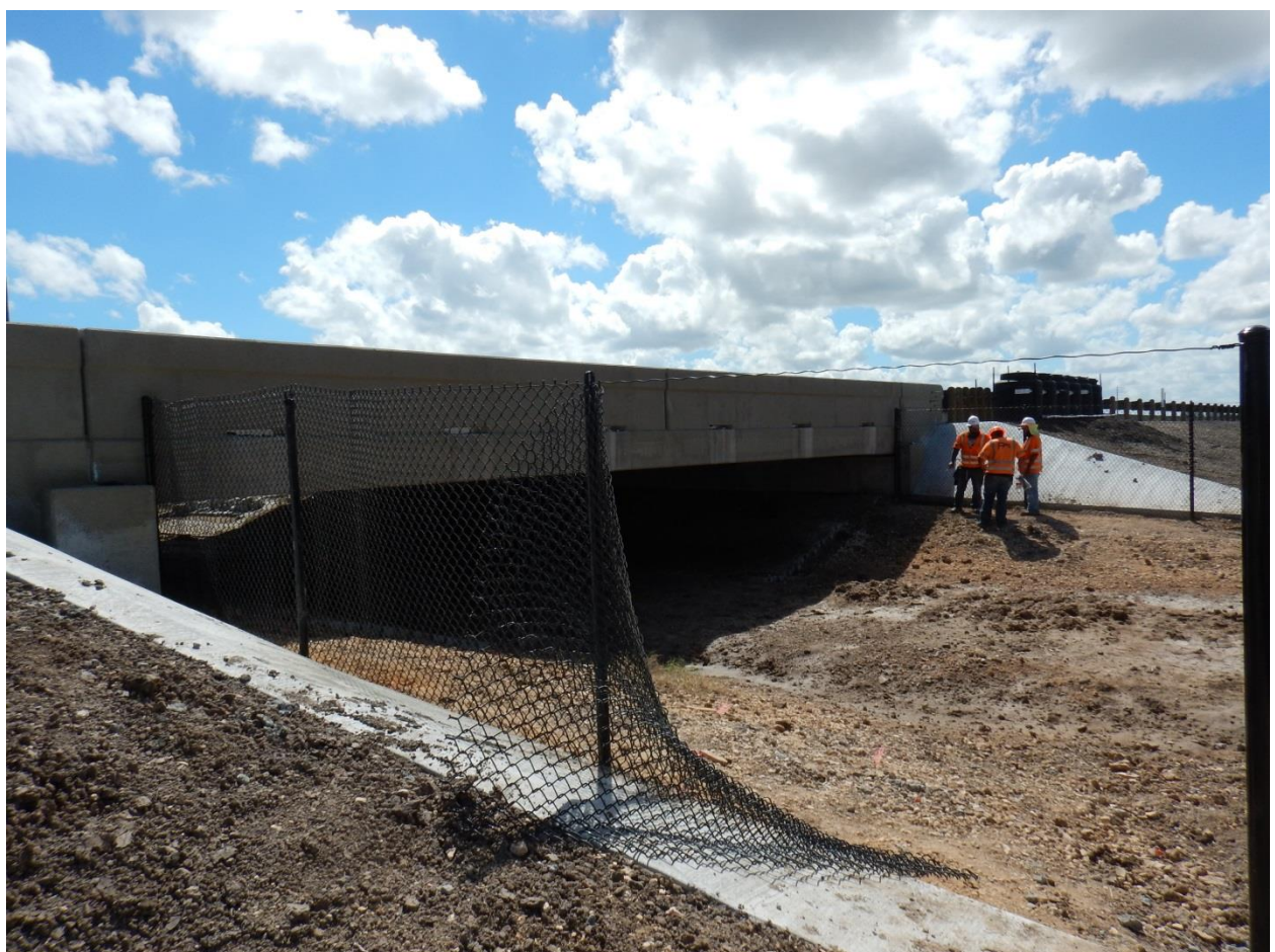
Figure H.13: Wildlife Crossing #3 "Half Bridge" Under Construction
