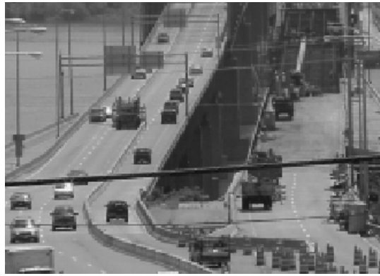
Figure 10. Movable Barrier in Use on McClugage Bridge (30)
