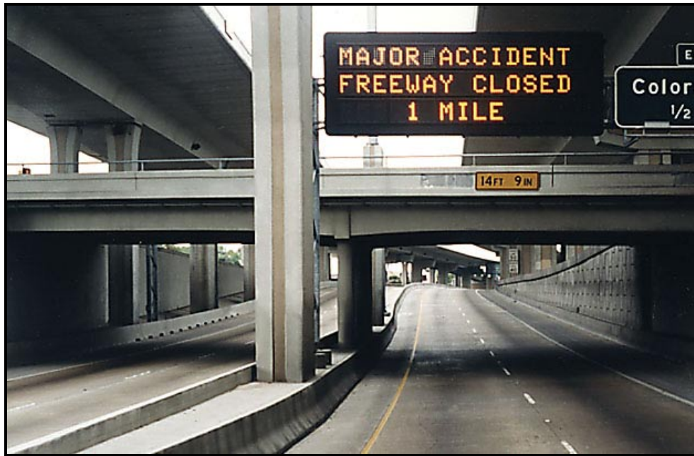
Figure 5. TransGuide System Dynamic Message Sign (23)
