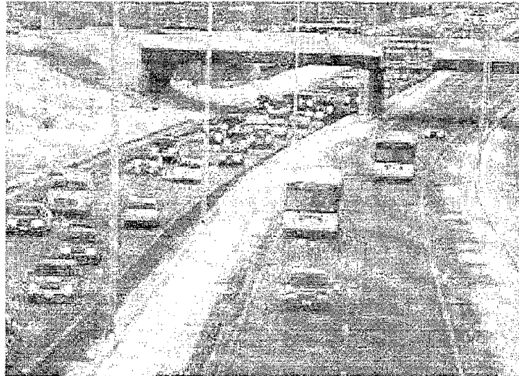
Figure 9. Reversible HOV Lane in the Center of I-394 in Minneapolis (41).
