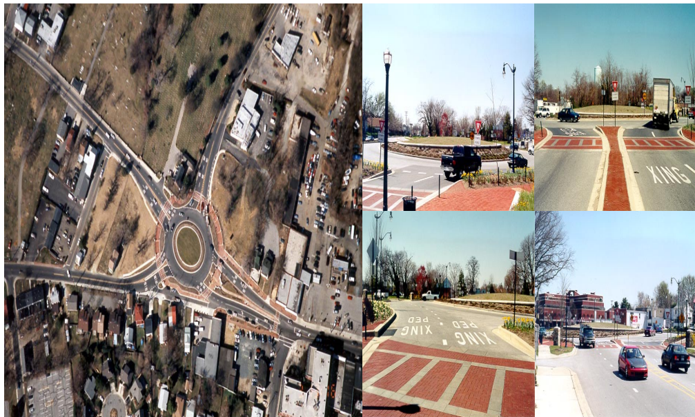
Figure 6. “After” Pictures - The Annapolis Westgate Circle Roundabout
