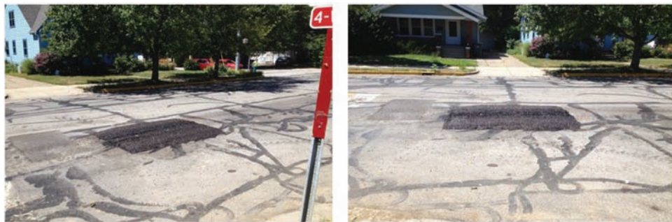
Figure 1.2 Example of a poorly performing utility cut. (Courtesy of Dr. Tommy Nantung and Dr. Jusang Lee, August 2015.)
