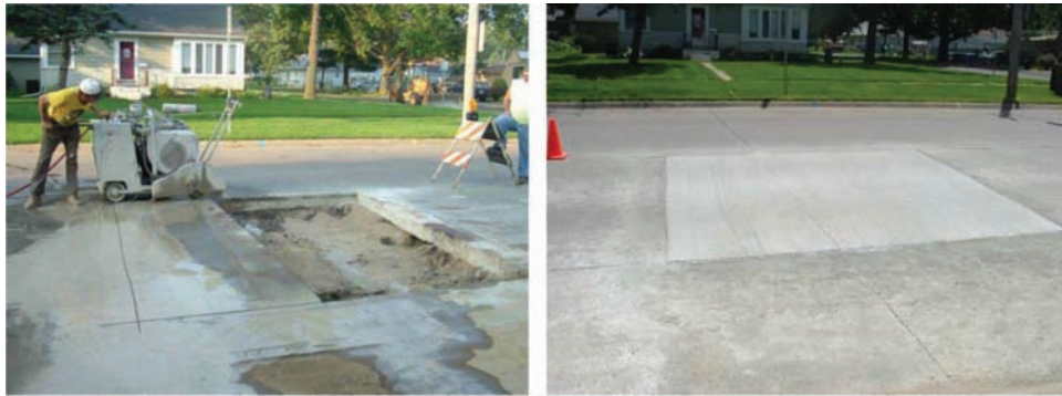
Figure 1.1 Example of a utility cut repair operation on a concrete pavement (Schaefer 2005).
