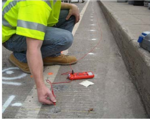
Figure 17. Continuity Test
