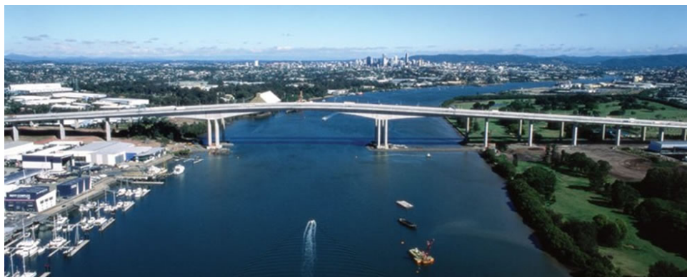
Figure 48. Gateway Upgrade Project (Gateway Upgrade Project, 2017)
