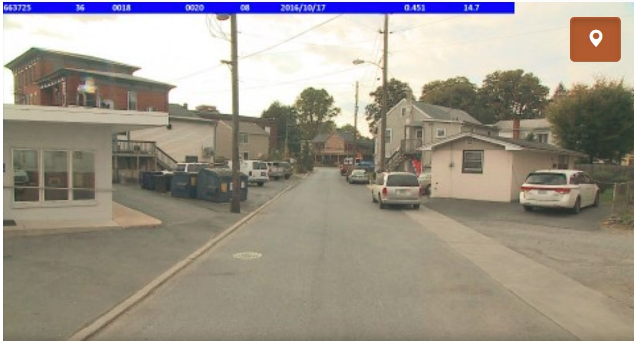
Figure 11. Example of sidewalk without curb (County 36, Route 18, Segment 20)
