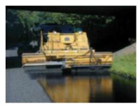
Figure 4. Chip seal application (left) (Crawford & Luce 2007) and thin HMA overlay placement (right) (courtesy of Suit-Kote Corporation).
