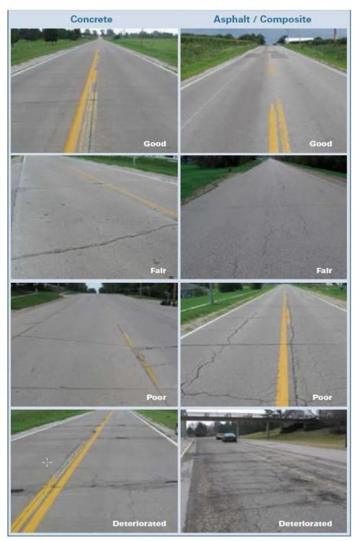
Figure 18. Example illustrations of overall pavement condition (Harrington and Fick 2014).
