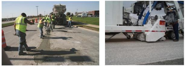
Figure 7. Partial-depth repair (left) and diamond grinding (right) (Smith et al. 2014).
