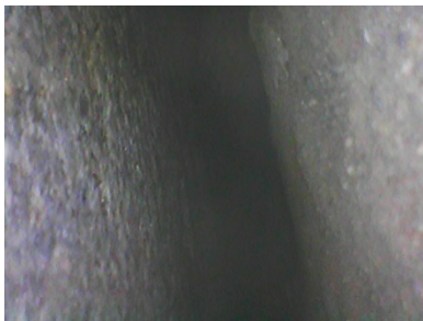
Figure 5-12: Boroscope view of gaps in non-grouted and deteriorated retaining walls by ME-concrete
