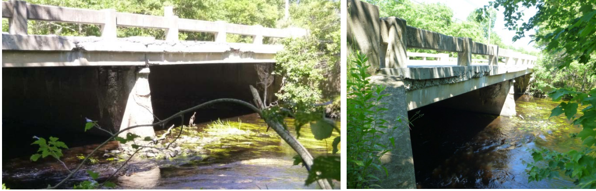
Figure 5-86: Deteriorated concrete bridge selected in RI (RI-precast_concrete_2)
