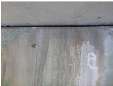
Figure 5-82: Staining of unidentified causation between the girders and where the girders and abutment meet in RI-precast_concrete
