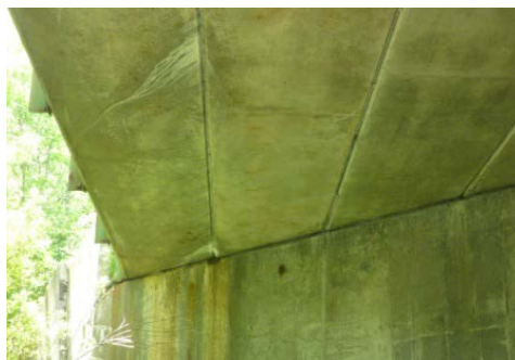
Figure 5-41: Staining of unspecified causation from gaps under beams at MA-precast_concrete_2
