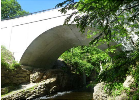
Figure 5-105: Concrete arch bridge selected in VT (VT-concrete_arch)
