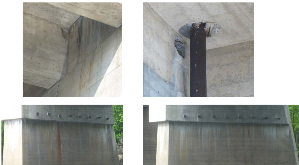
Figure 5-14: Staining of unknown causation at ME-concrete
