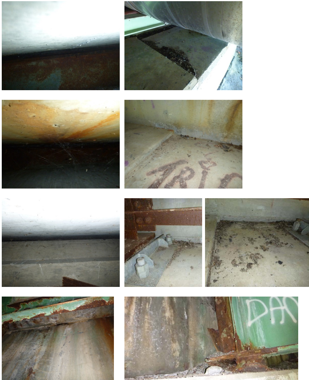
Figure 3-9: View into the expansion joint (left), and the material found below (right)
