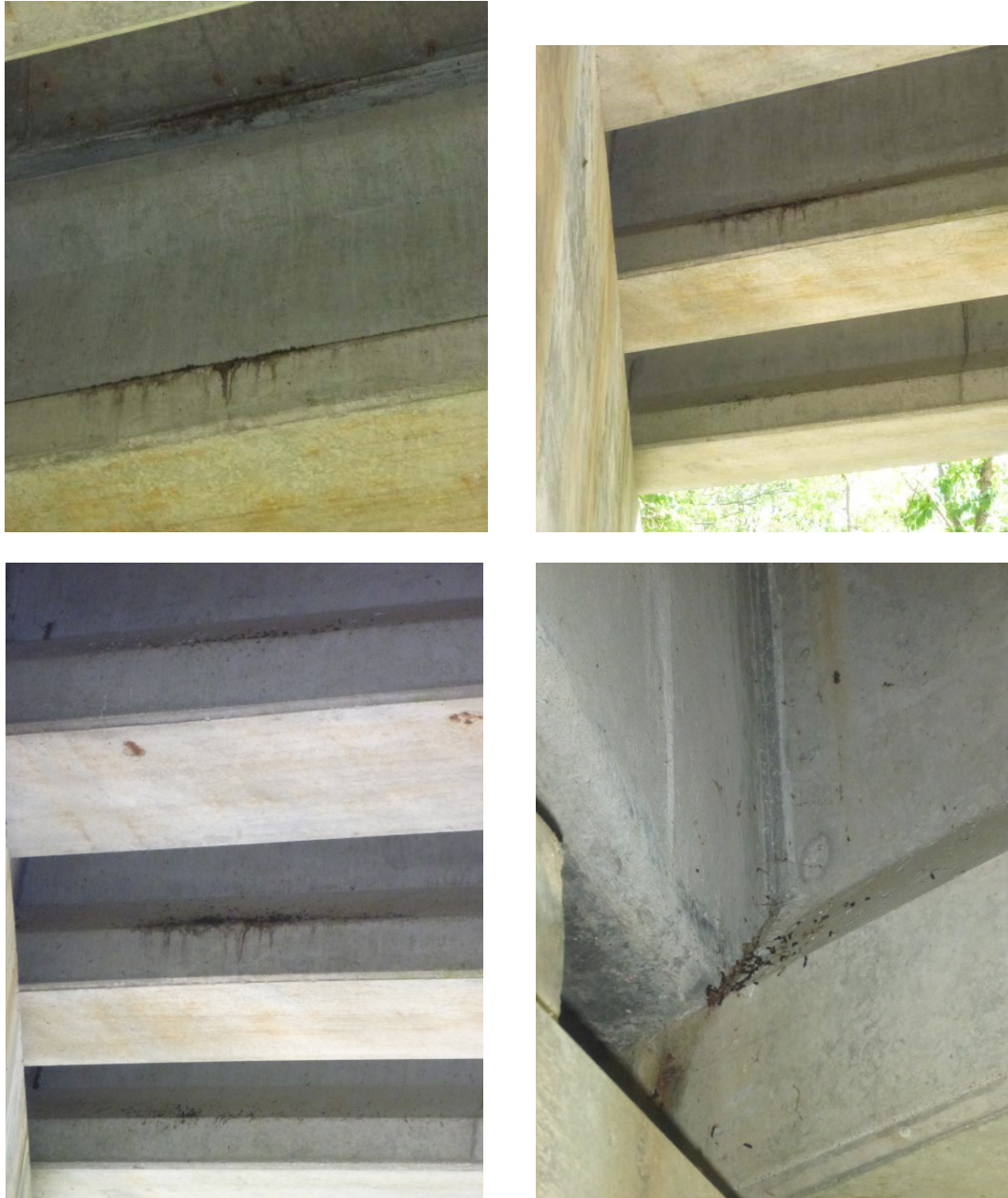
Figure 4-12: Staining evidence of roosting on bridge girders at bridge in Washington County, RI
