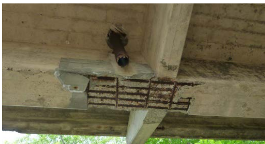
Figure 5-10: Downspouts at ME-concrete
