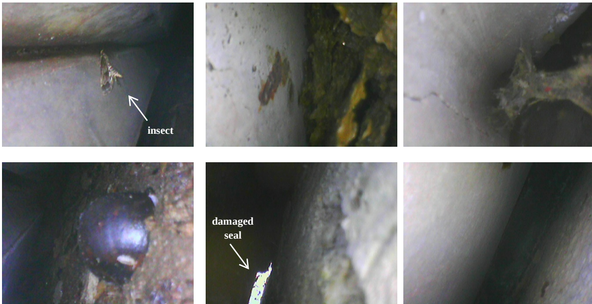
Figure 5-83: Boroscope view between girders and between girders and the abutment at RI-precast_concrete showing insects, debris, structural components, sealant damage, and clean gaps
