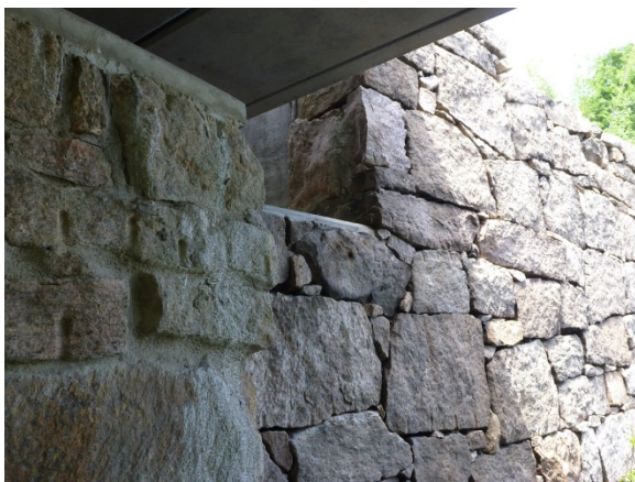
Figure 3-15: Construction with grouted stonework and non-grouted stonework (left and right sections of photo)
