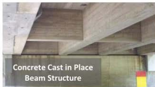
Concrete Cast in Place Slab Structure
