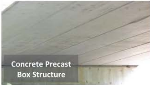
Concrete Precast Box Structure
