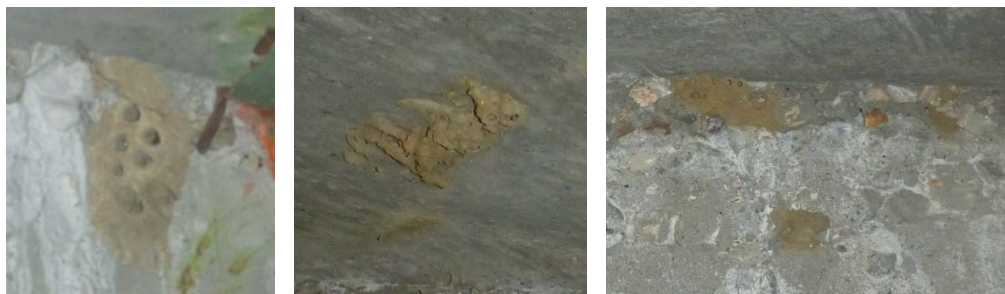
Figure 5-52: Mud-Dauber's nests observed at MA-steel
