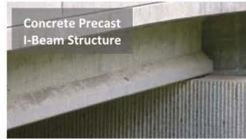
Concrete Precast Beam Structure
