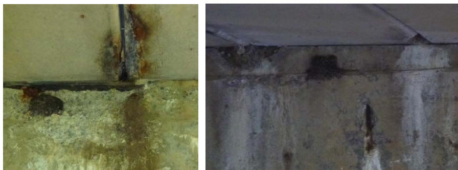
Figure 5-89: Bird's nests observed at RI-precast_concrete_2
