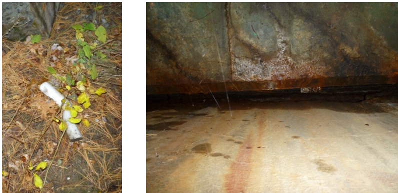
Figure 5-99: Insulation (left) that has fallen out of an expansion joint (right) at RI-steel_2
