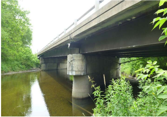
Figure 5-117: Steel construction bridge selected in VT (VT-steel)
