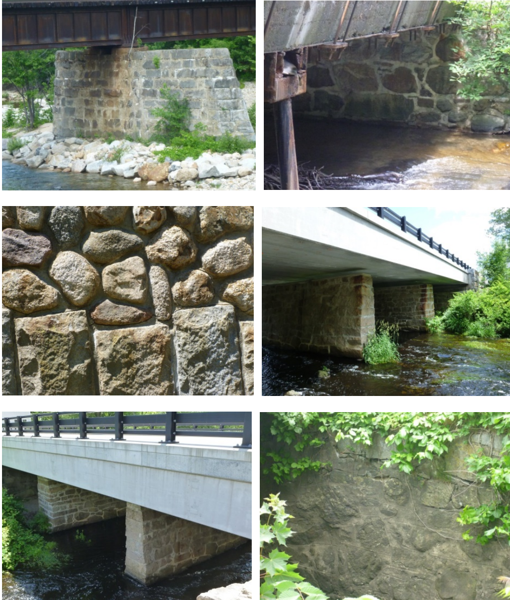
Figure 3-17: Grouted stonework does not create suitable roosting crevices and locations
