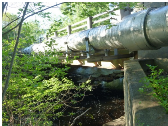
Figure 5-92: Pipes around RI-steel bridge
