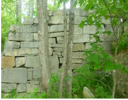
Figure 5-11: Rock partial retaining wall adjacent to the abutment at ME-concrete
