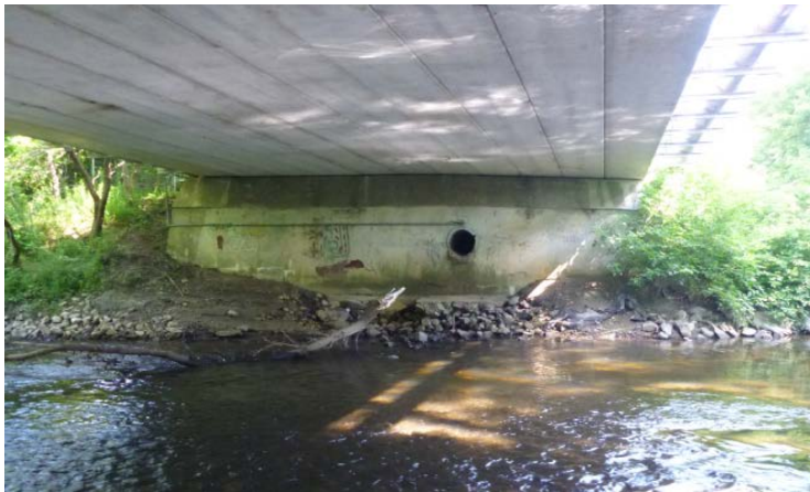
Figure 5-35: Precast concrete bridge selected in MA (MA-precast_concrete)
