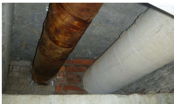
Figure 5-29: Pipes observed at MA-concrete
