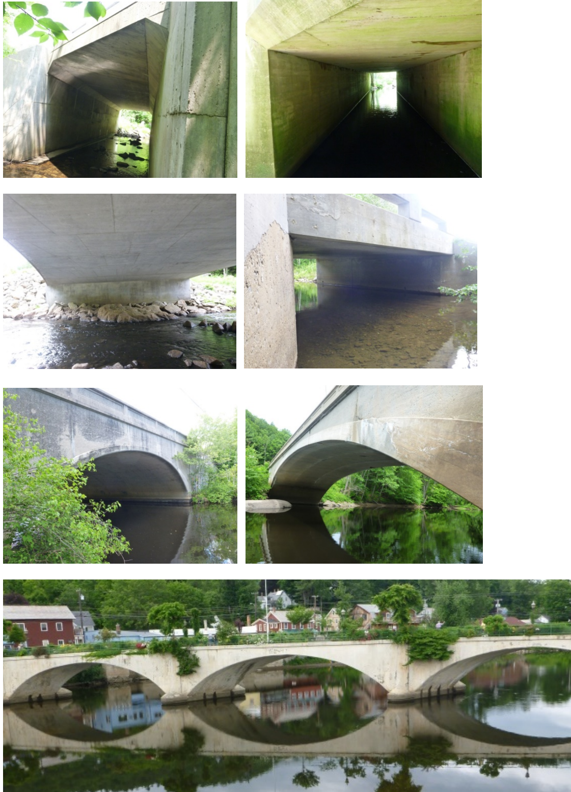
Figure 3-20: Bridges with only smooth surfaces lacking roosting locations
