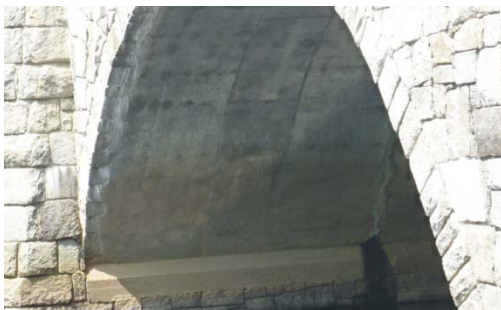
Figure 5-57: Smooth inside arch in NH-concrete_arch
