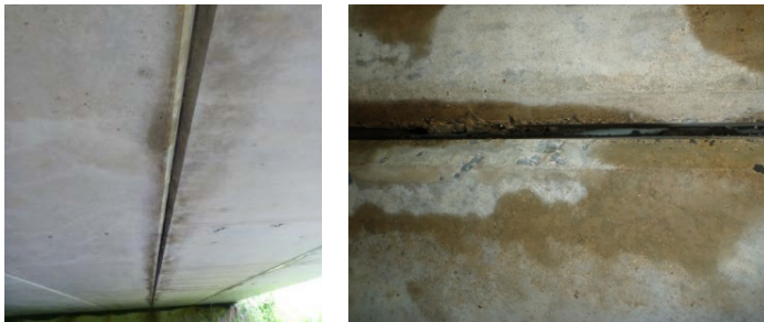
Figure 5-2: Gaps between girders in CT-concrete
