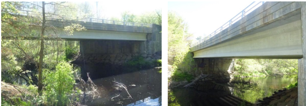
Figure 5-72: Concrete bridge selected in RI (RI-concrete)
