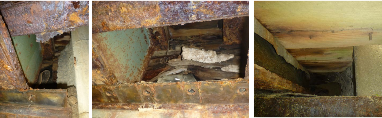
Figure 5-21: Potential roosts by the abutments in ME-steel/wood
