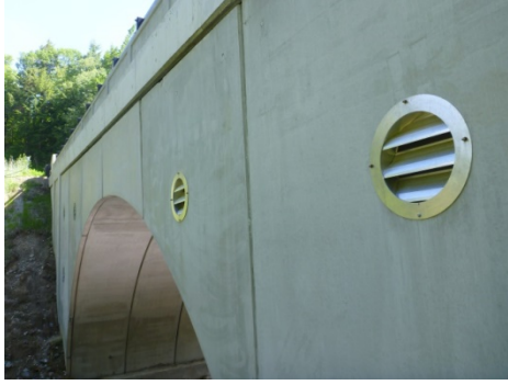
Figure 5-109: Vents on the opposite side of VT-concrete_arch
