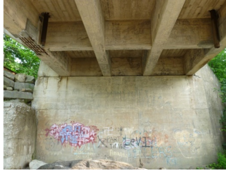
Figure 5-11: Rock partial retaining wall adjacent to the abutment at ME-concrete
