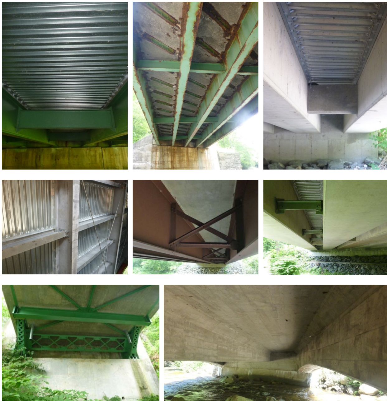
Figure 3-18: Bridge deck construction that does not create suitable roosting crevices and locations
