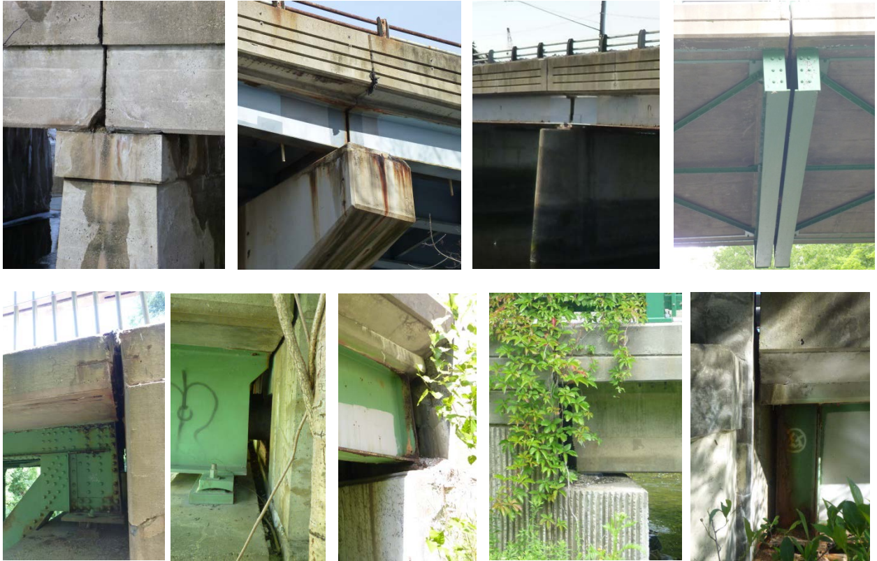
Figure 3-8: Expansion joints
