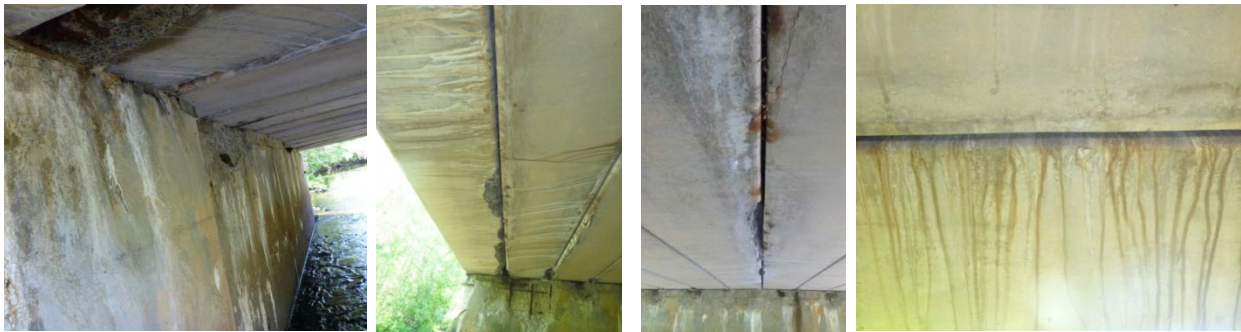
Figure 5-87: Cracks and crevices that can be potential roost sites in RI-precast_concrete_2
