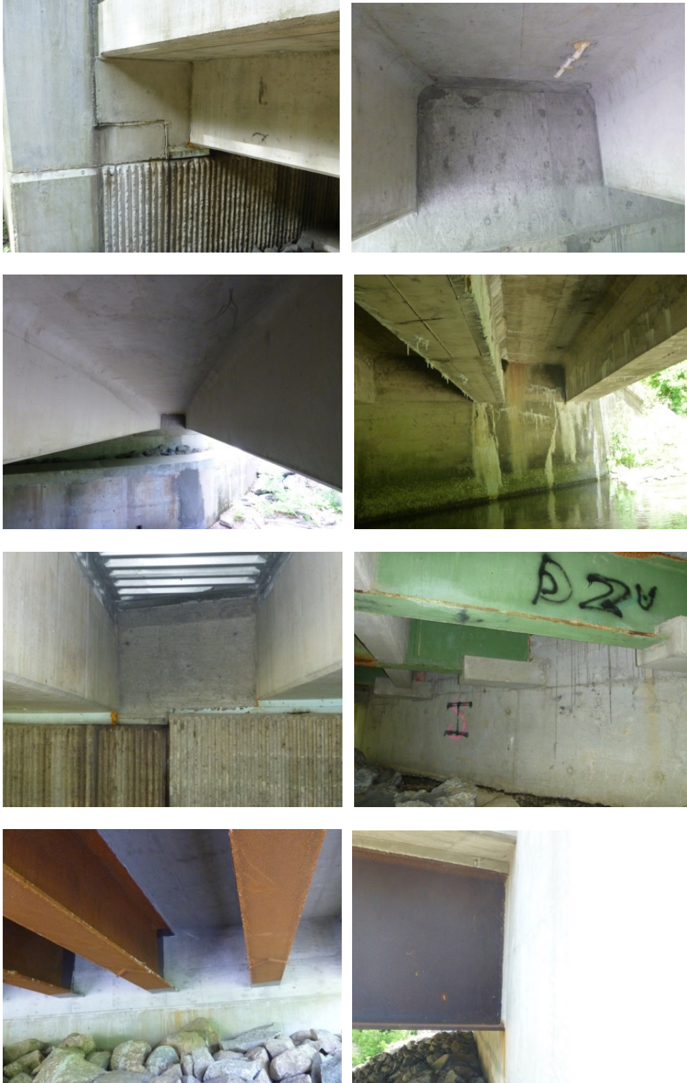
Figure 3-19: Bridges with integral abutments
