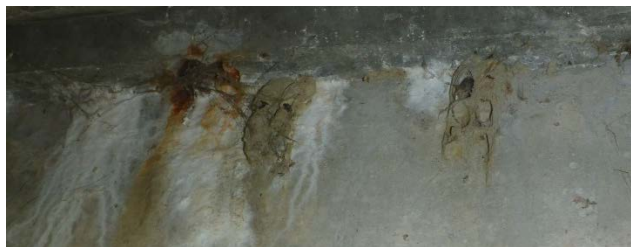
Figure 5-6: Mud-Dauber's nests observed on CT-concrete
