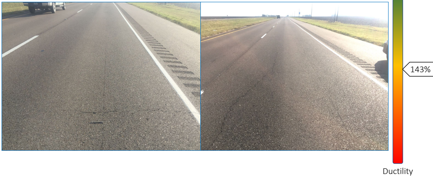
Section #15: 4 years Photo and coring from Nov. 2019 as cracks are beginning to emerge
