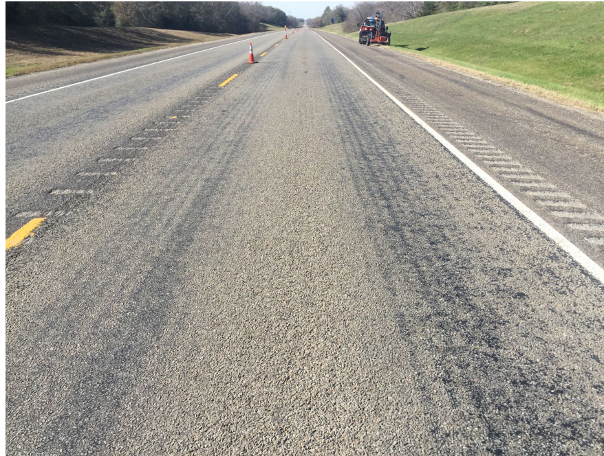
Section #5: 5 years Photo and coring from Dec. 2019 after seal coat was placed
