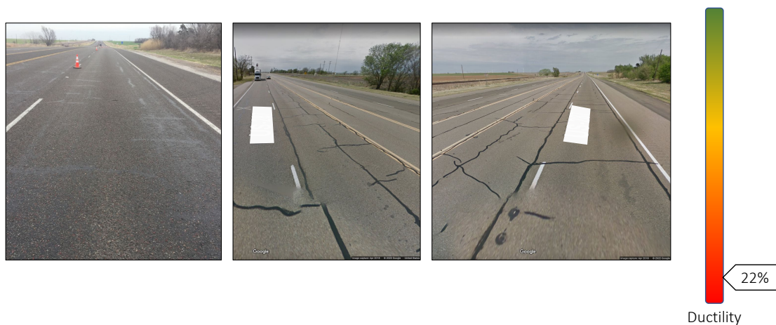
Figure 5.10. Section #19, 7 years at the time of coring, left - phot and coring from March 2020 after a recent seal coat showing some bleed through cracks, middle and right - Google street view from April 2018 before the seal coat was placed showing extensive cracking
