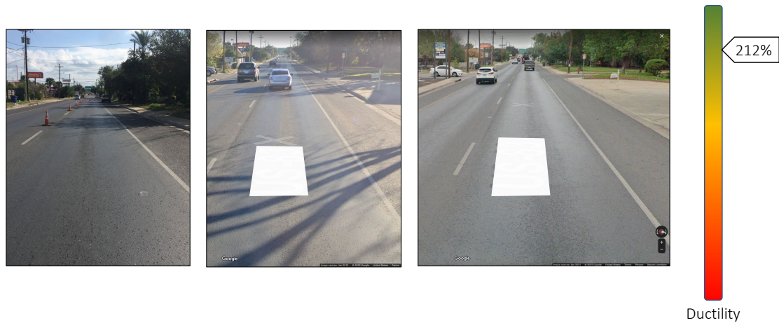
Figure 5.6. Section #7, 7 years at the time of coring, left - photo and coring from November 2021, middle and right - Google street views from January 2019 and April 2021 prior to coring showing no cracking over time
