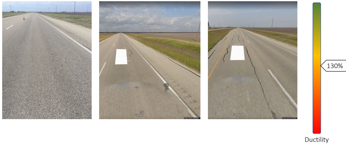
Figure 5.8. Section #17, 6 years at the time of coring, left - photo and coring from November 2019 when there were no apparent surface cracks, Middle and Right - Google street view from December 2021 showing cracks along the wheel path that have already been sealed
