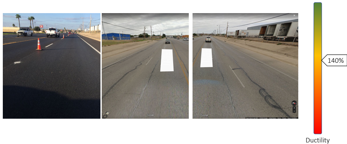
Figure 5.7. Section #6, 7 years at the time of coring, left - photo and coring from November 2021 after a recent overlay, Middle and Right - Google street view from April 2021 before the overlay was placed showing cracking along the wheel path
