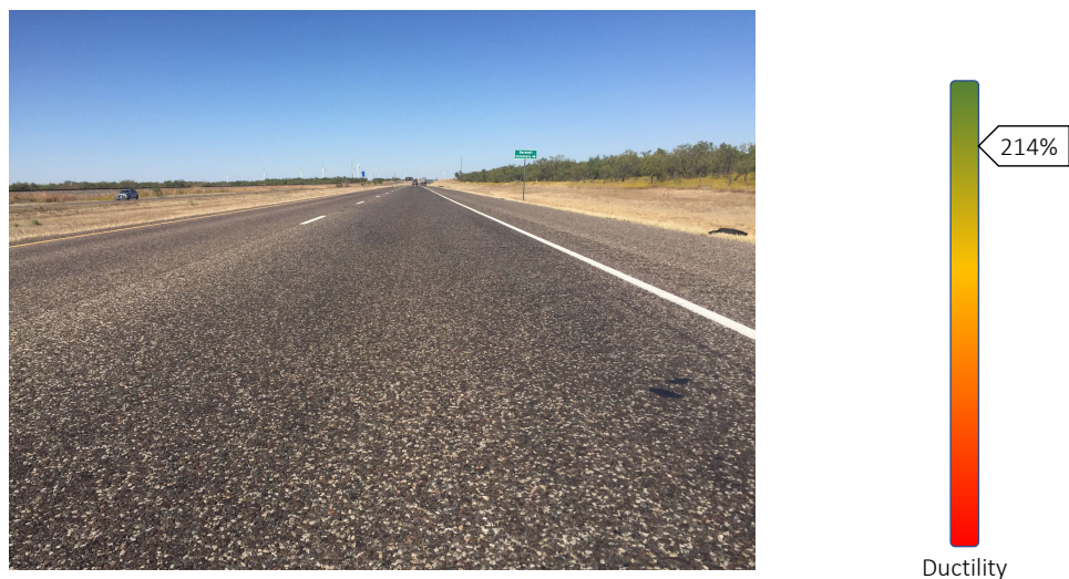
Figure 5.5. Section #18, 7 years at the time of coring, photo and coring from October 2019, no cracking was observed at the time of coring
