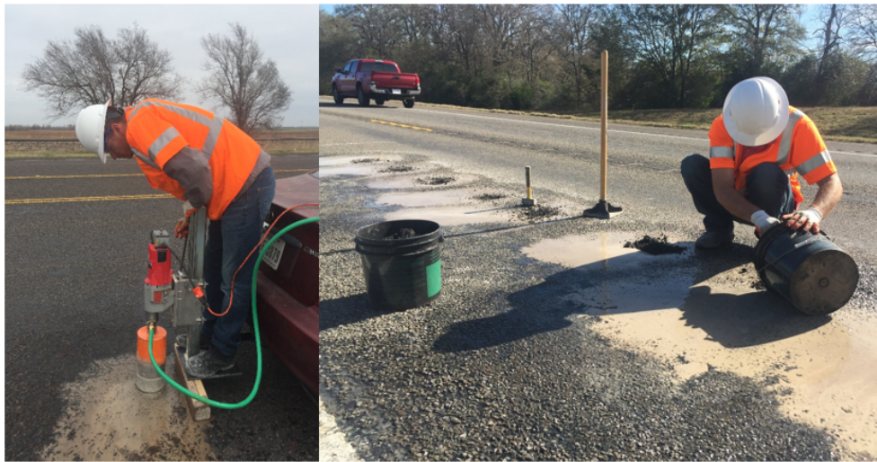
Figure 2.2. Field coring and patching.
