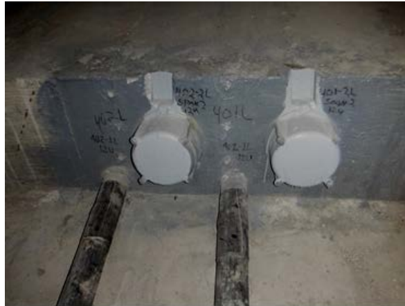
Photograph 2- Anchorage blocks at center of spans
