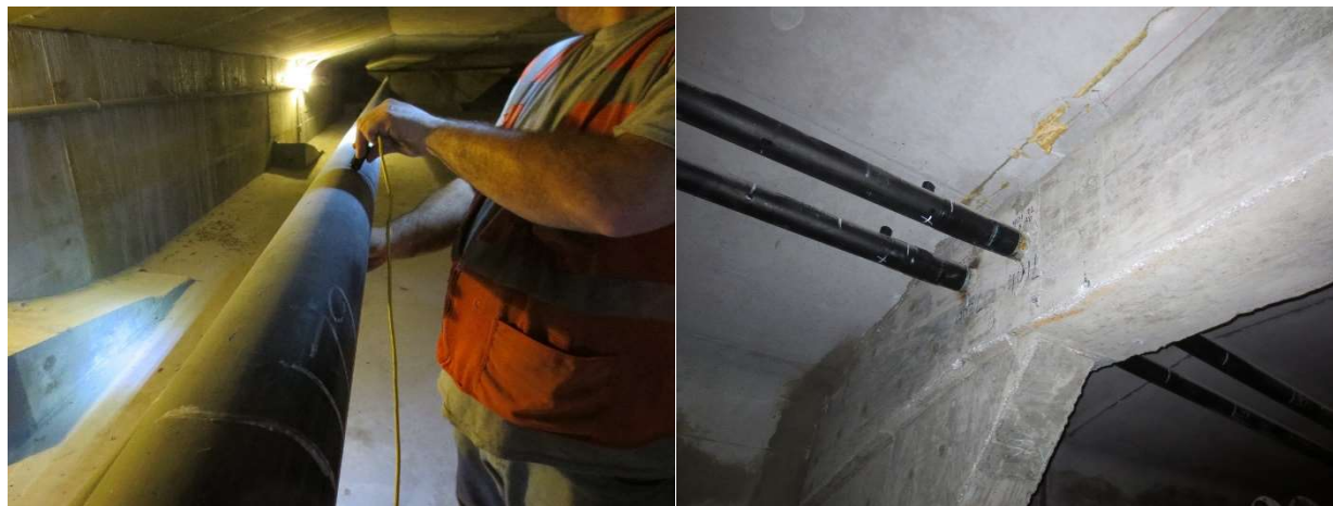
Figure 2-1: Measurements on tendon (left) and high elevation tendon spans (right).
