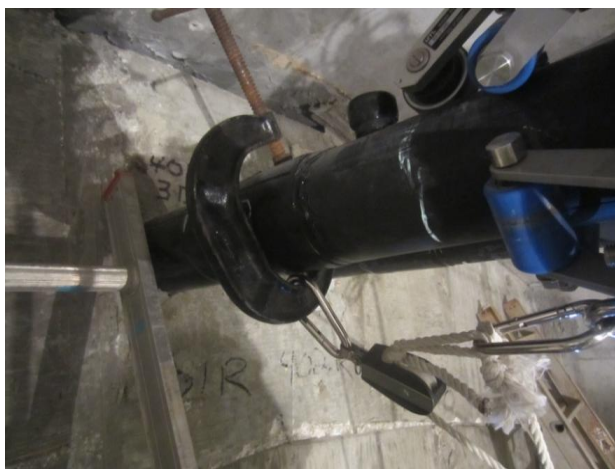
Figure 25. Installing a steel clamp and a pulley.
