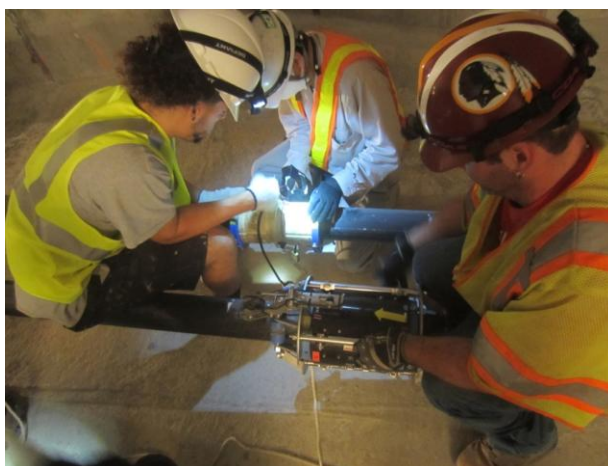
Figure 26. Installation of two magnetizers on the inclined sections at low elevation.
