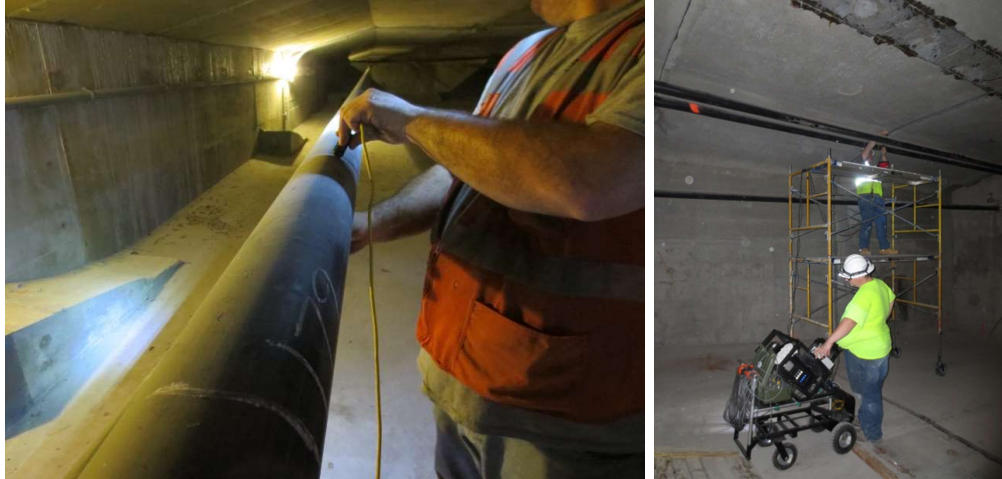
Figure 4-1: Ultrasonic/sonic testing on external PT tendons.
