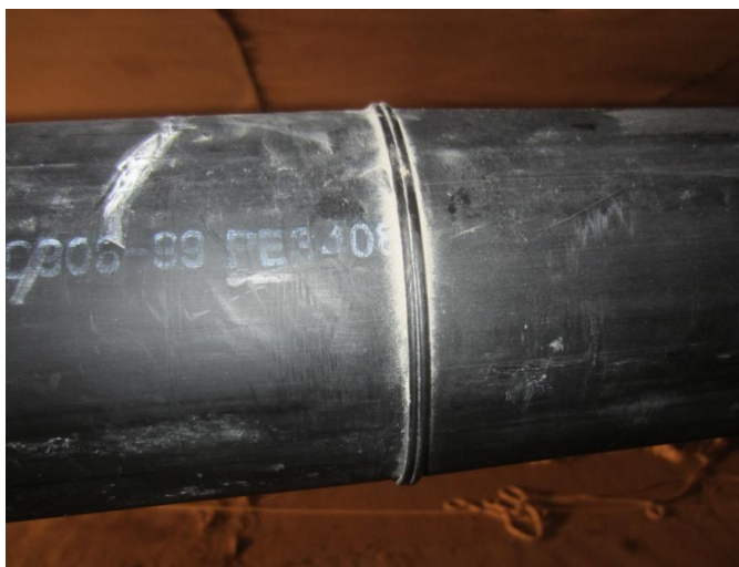
Figure 32. Extruded HDPE welding joint.
