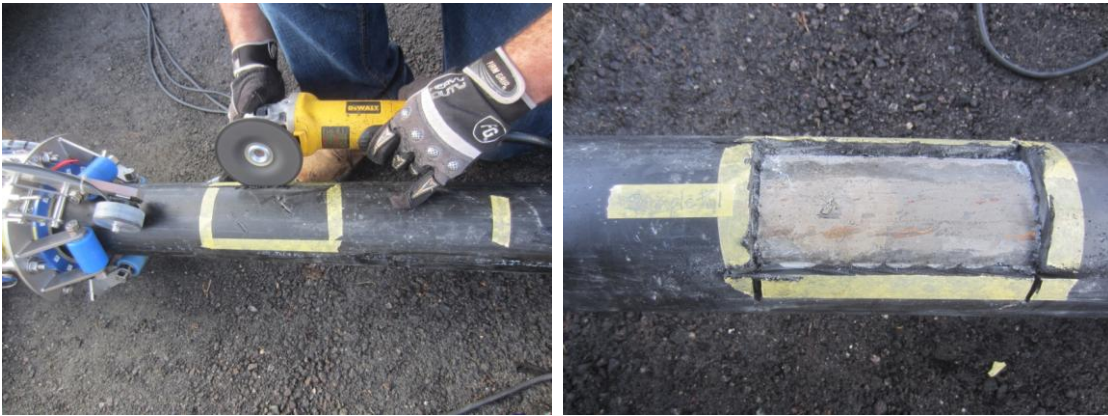
Figure 12. Making a 6 x 3 inches duct opening (left) and as-exposed grout condition (right).
