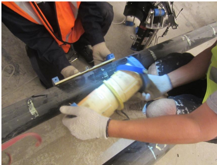
Figure 6. Installing two half-split sensor holder pieces on a tendon.
