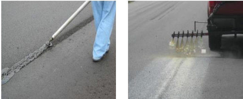
Figure 2.9: Joint adhesive and sealant construction (Williams 2011)
