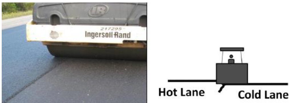
Figure 2.3: “Cold Roll Rolling Pattern” on asphalt pavement. (Williams 2011).
