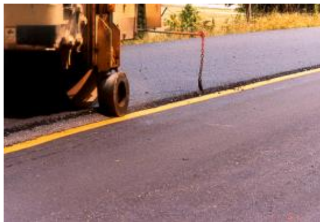
Figure 2.5: Edge restraint construction (Fleckstein et al. 2002)
