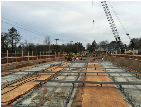
Figure 1 – Westbound bridge overpass, Union Street, Bangor (2014-12-14)
