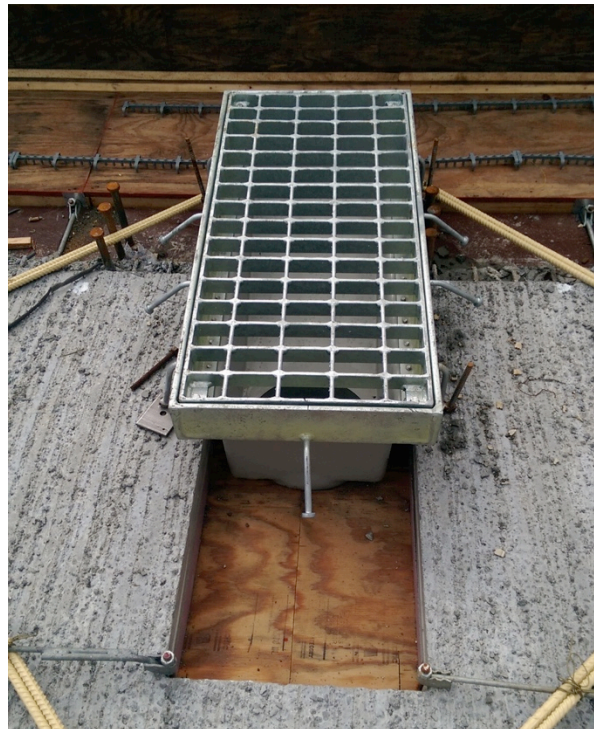
Figure 29 - Drain in place prior to rebar placement
