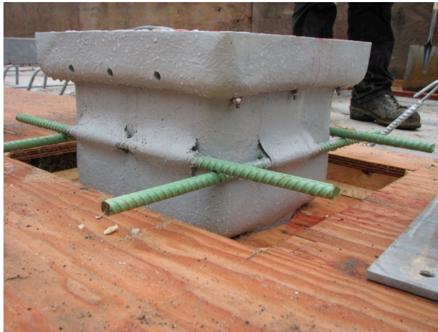
Figure 8 – Drain side holes and rebar (2014-12-14)
