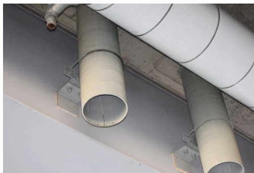
Figure 21 – Drain pipes in the westbound bridge overpass (2015-10-05)
