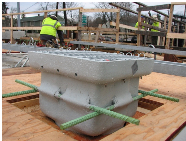
Figure 10 - Drain and formwork (2014-12-14)
