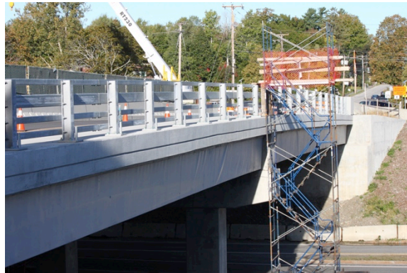
Figure 20 - Westbound bridge overpass after construction (2015-10-05)
