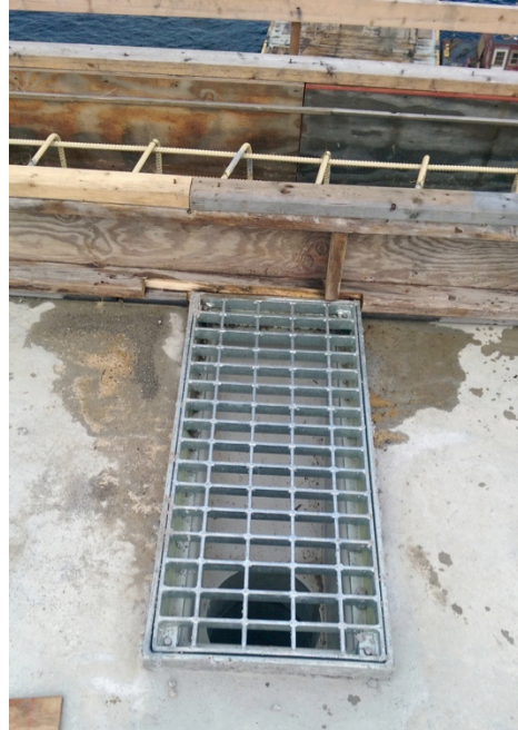
Figure 30 - Drain after concrete placement
