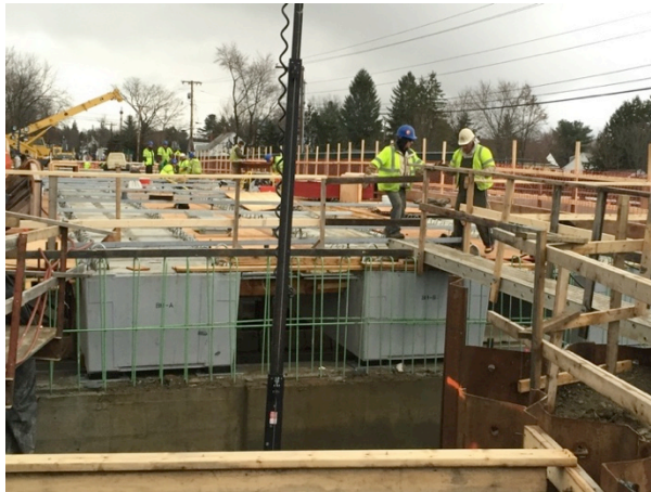
Figure 2 – HCB beams of the westbound bridge overpass (2014-12-14)
