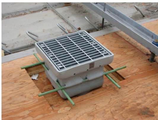
Figure 3 – Drains installed over formwork (2014-12-14)
