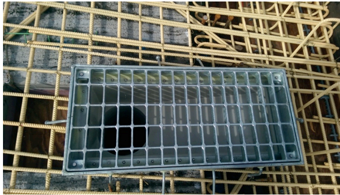
Figure 27 - Drain and grate at another location prior to concrete placement
