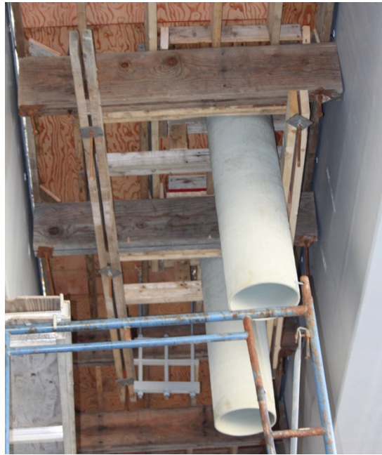
Figure 19 – Drain pipe prior to concrete placement (2015-10-05)
