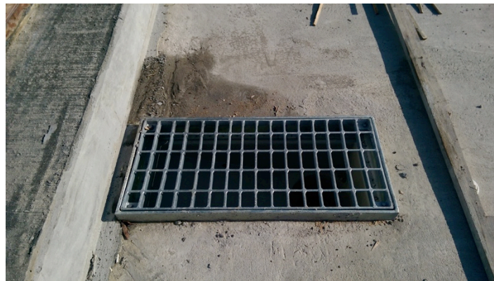
Figure 31 - Drain in place after concrete placement
