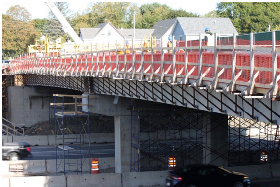
Figure 16 - Eastbound bridge overpass during construction (2015-10-05)
