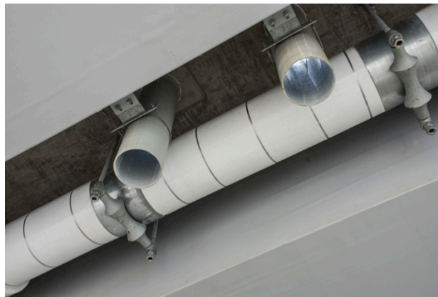
Figure 15 – Drain pipes and attachments (2015-06-03)
