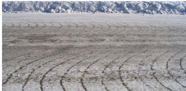
Figure 2.2. Deicing operation using pre-wetted sand by hot water (Perchanok et al., 2010)
