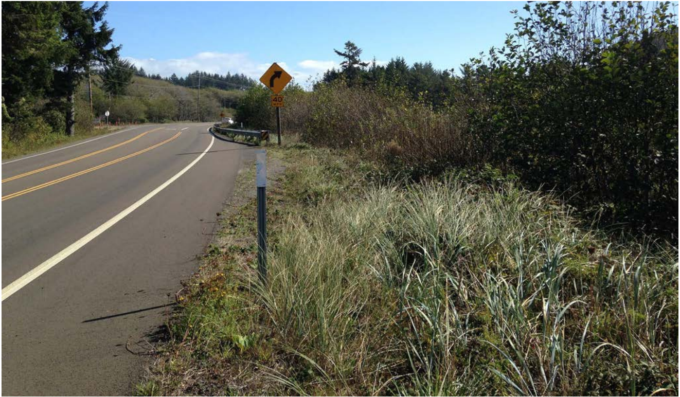
US 101 at the Ona Beach study site; much of this low-lying area is vegetated with willows and wetland plants. Credit: ODOT.
