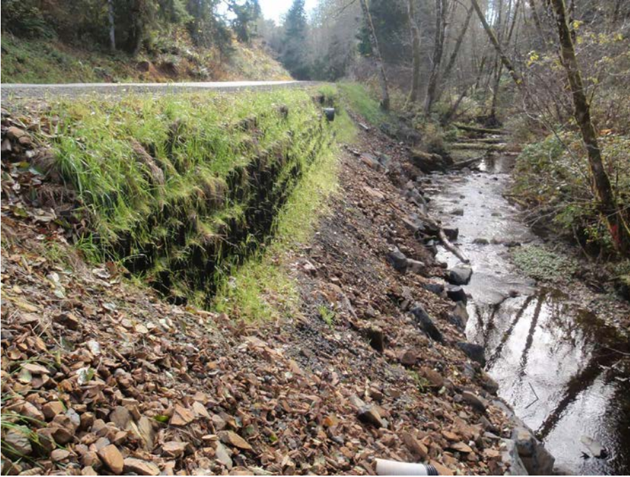
Vegetated MSE slope. Credit: ODOT
