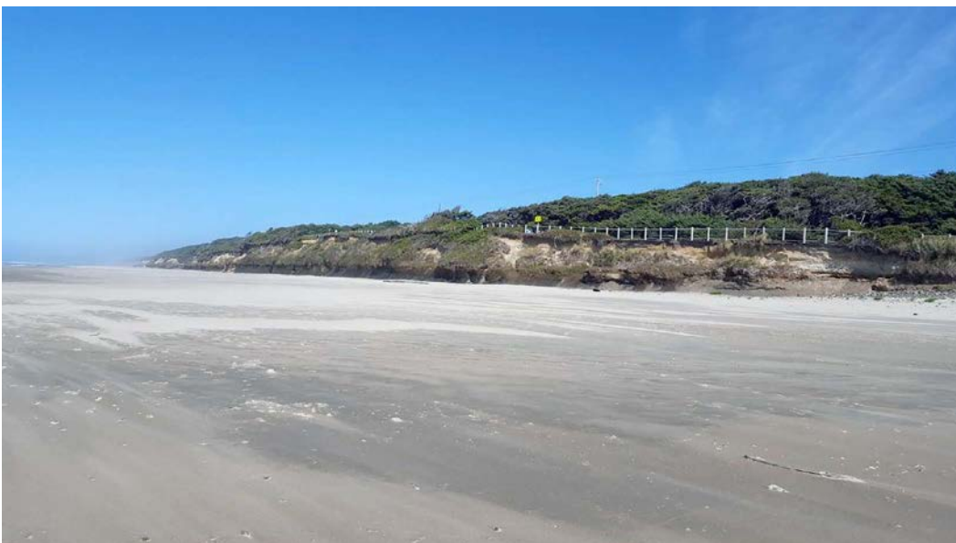
Active erosion of the coastal bluffs can be seen along the backshore at Lost Creek. Credit: ODOT.
