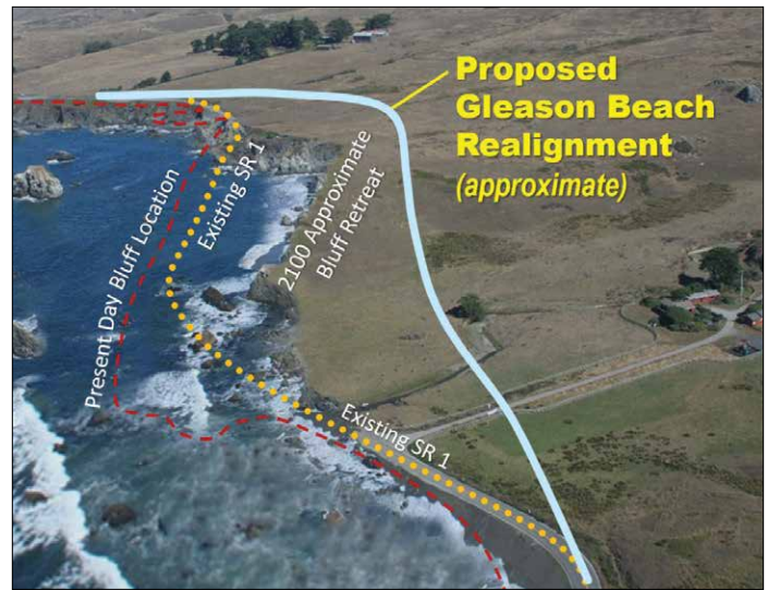
View of the present-day bluff location and projected 2100 approximate bluff retreat, which depicts the limit of the expected coastal erosion, as well as the proposed realignment. Photo: Google Earth with information from Caltrans District 4
