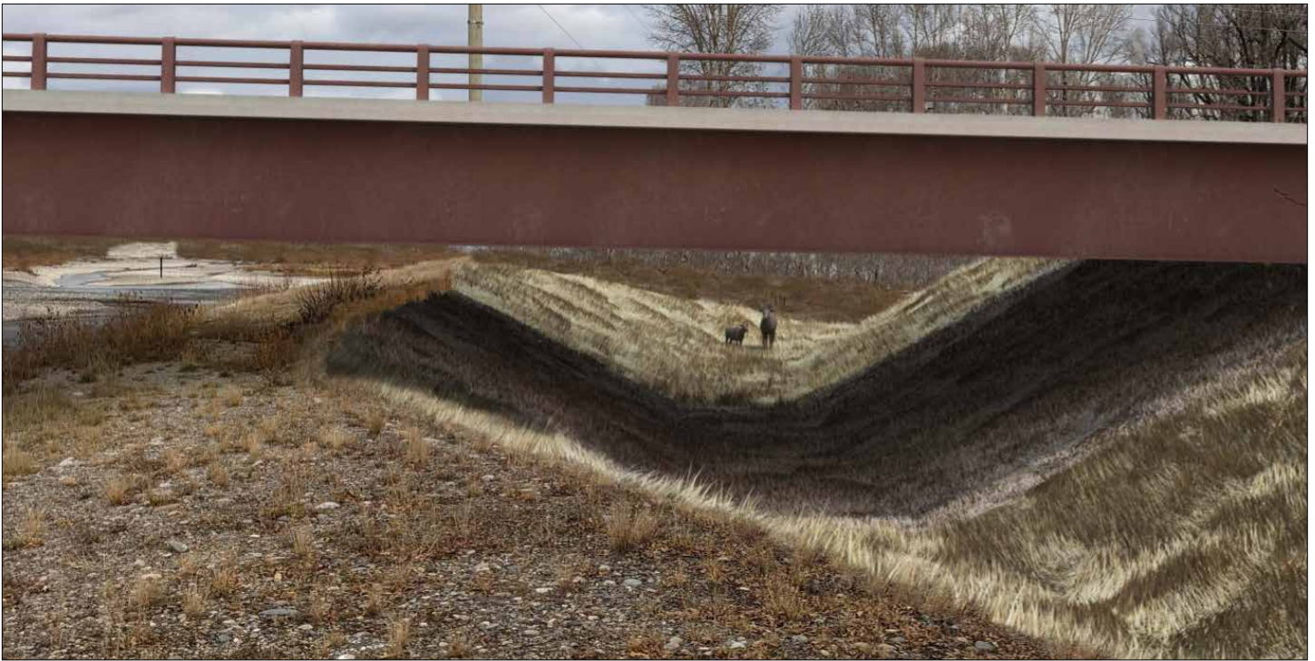
The Snake River Bridge Extension features a wildlife underpass and enhanced pathway that will help to address many challenges from wildlife-vehicle collisions to congestion. Photos: Wyoming Department of Transportation
