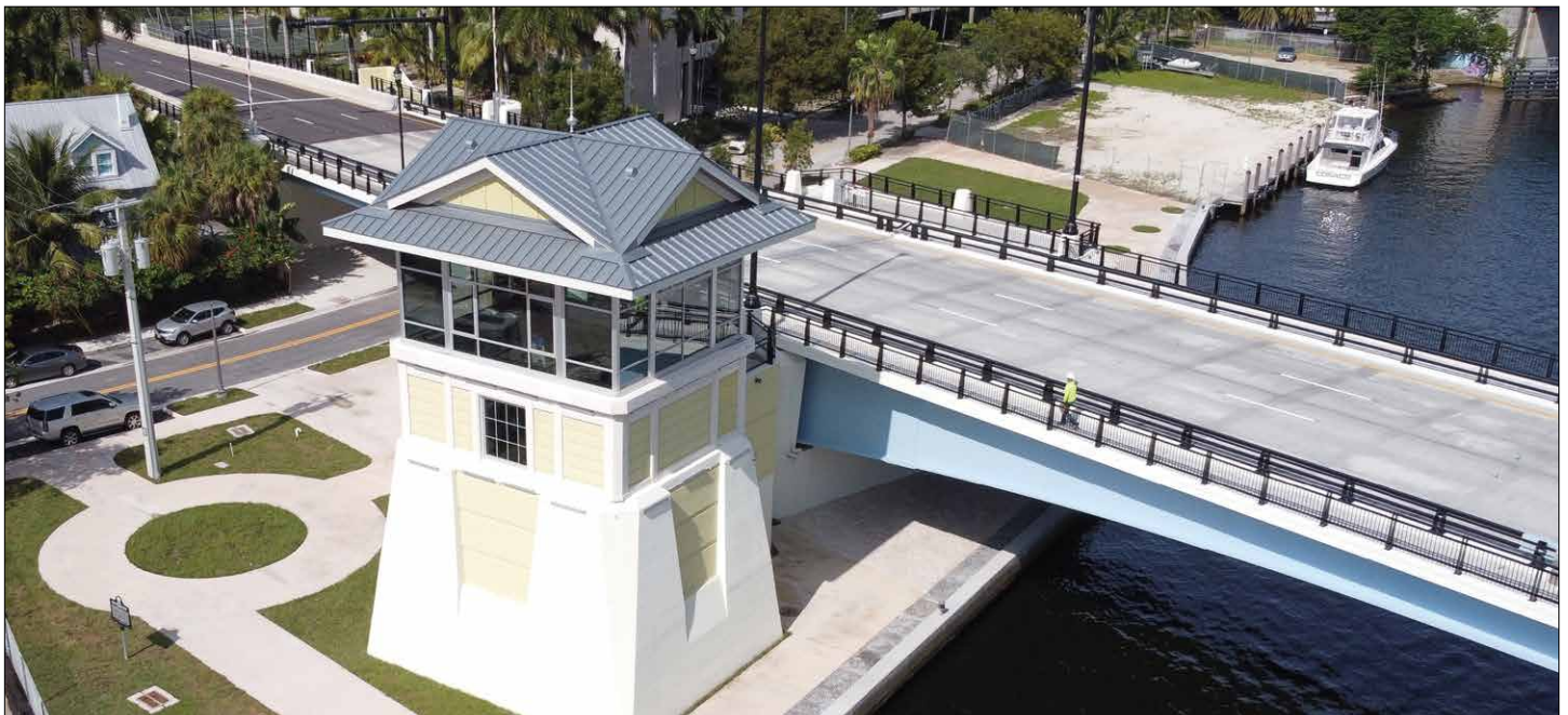
Looking northwest at completed bridge tender house and replacement bridge. Photo: Hardesty and Hanover, Inc.
