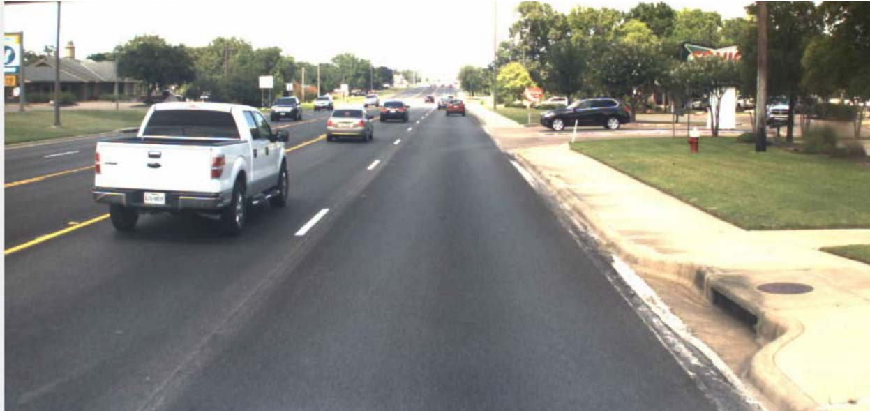
Figure 66. Urban Curb and Gutter Section Example.
