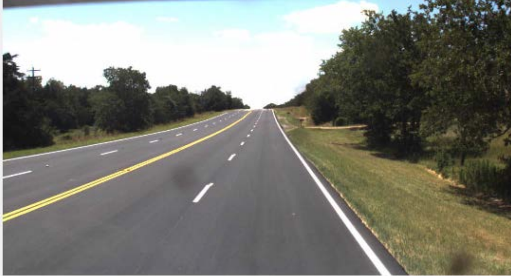
Figure 101. Spot Overlay on US 77.
