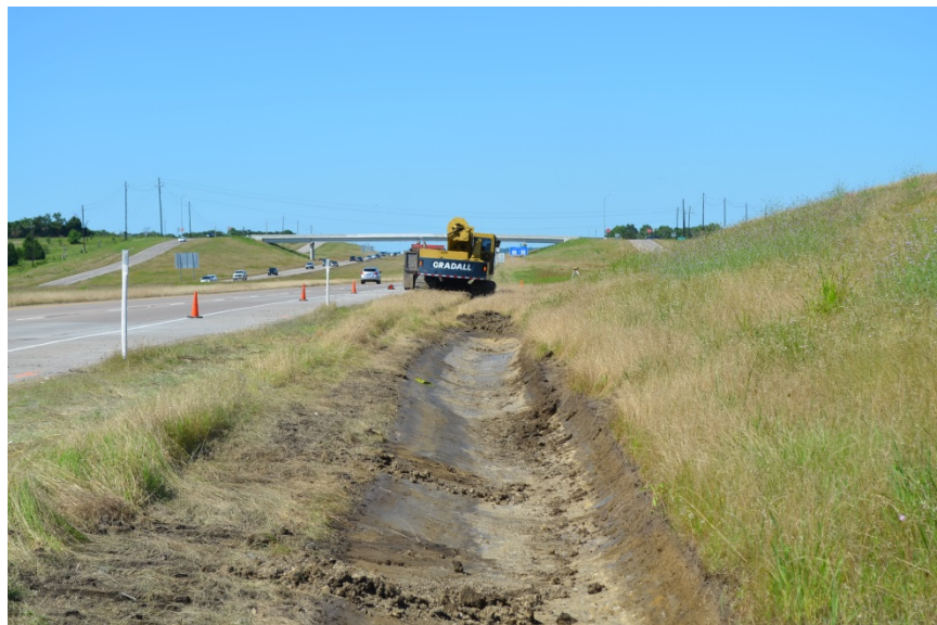
Figure 80. Ditch Grading Work along US 75.
