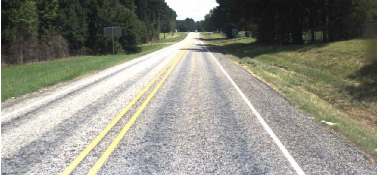
Figure 54. FM 2661 Widened Section North of SH 31.
