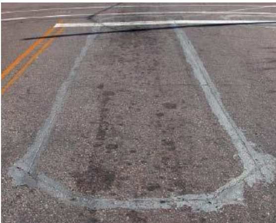
Figure 1.2.1 An example of inductive loop detector
