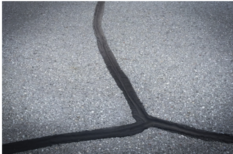
Figure 15. Good Overband Method (Courtesy of Roger Smith, 2021)
