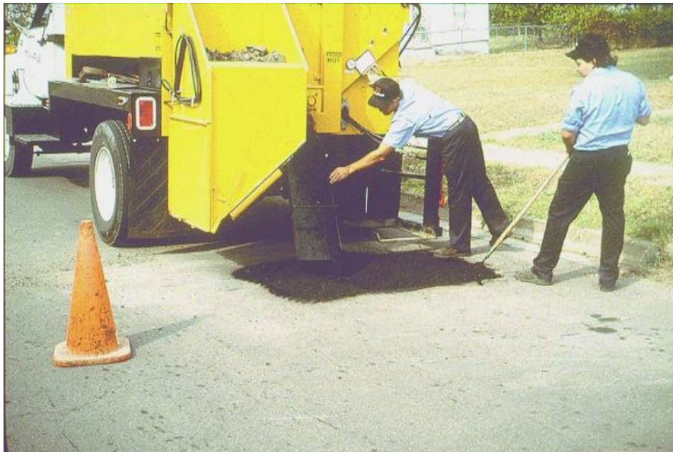
b. Unload Patching Material from Patching Truck
