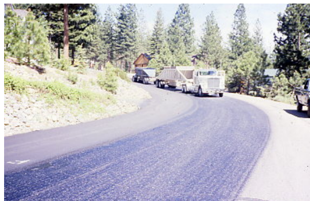
Figure 55. Sparse Tack Coat after Break
