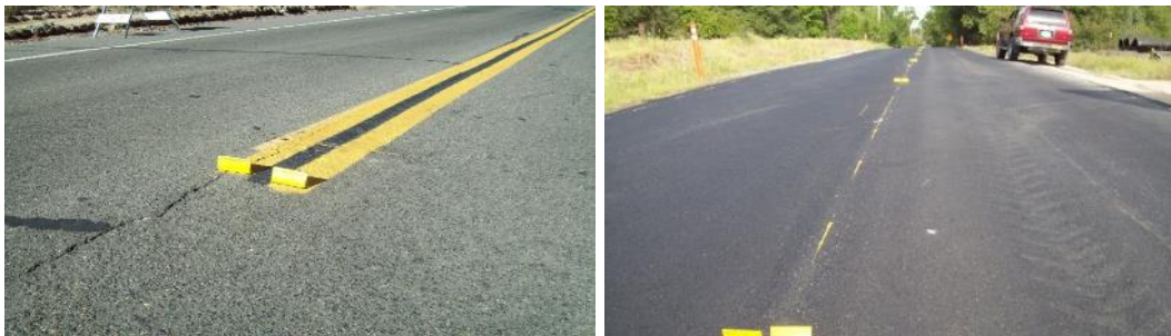
Figure 56. Temporary Lane Markers in Place Prior to Surface Treatment
