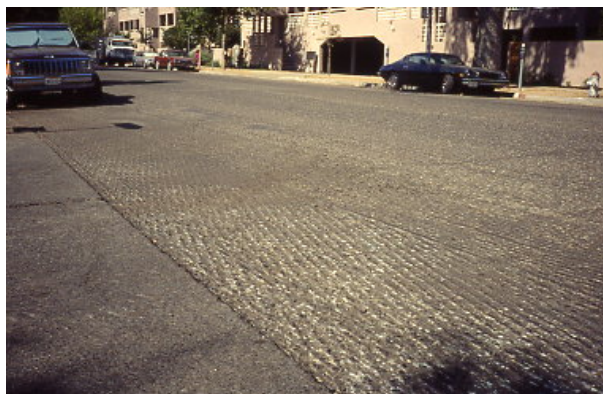
Figure 59. Milling of Entire Street to Reduce High Crown
