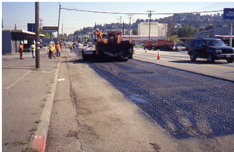
b. Paving HMA on a Tacked Surface
