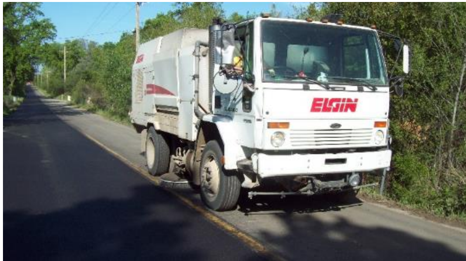
Figure 52. Sweeping Prior to Resurfacing
