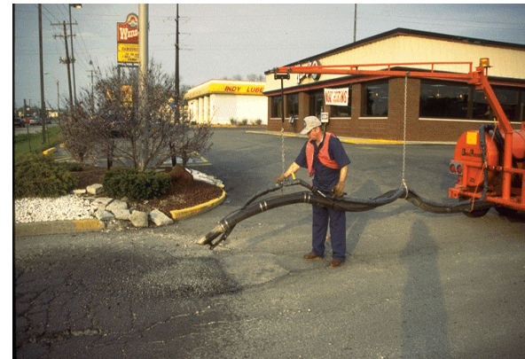
d) Application of Finish Coat of Aggregate
