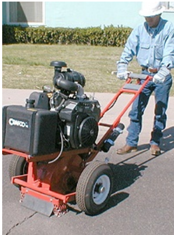
Figure 18. Routing to Create Crack Reservoir
