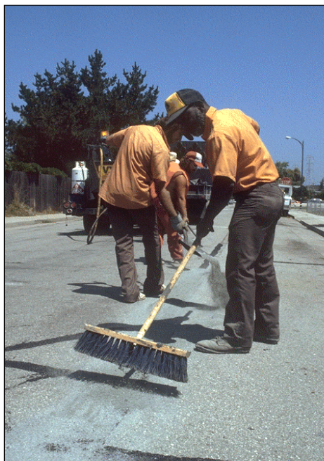
Figure 22. Brooming Blotter Coat over a Treated Crack
