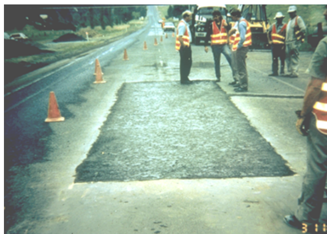
Figure 39. Completed Digout Patch using HMA (Caltrans MTAG, 2009)
