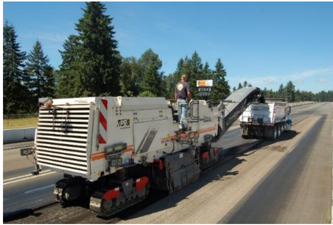
a. Milling Out the Distressed Area
