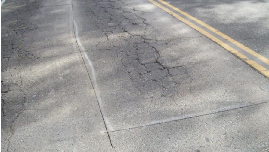
Figure 35. Marked Cut Lines for Small Digout
