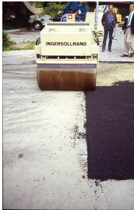
Figure 38. No Vibratory Rolling on Surrounding Good Pavement
