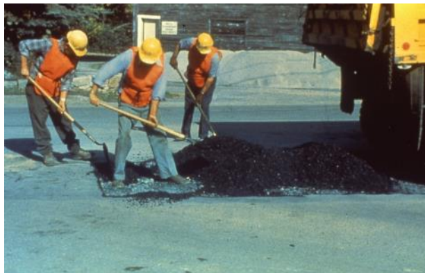
Figure 37. Spreading Patch Material into the Digout
