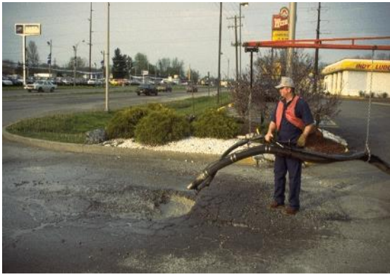
a) Site Preparation
