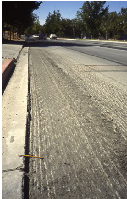
Figure 57. Edge Milling/Key Cutting
