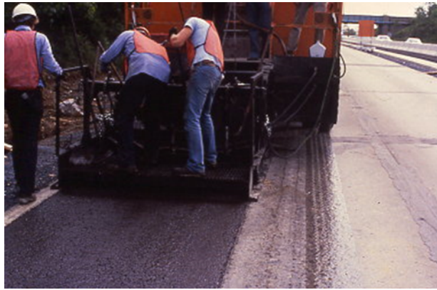
Figure 64. Rut Filling Using Microsurfacing Rut Box
