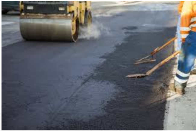
Figure 50. Rolling of a Skin Patched Area
