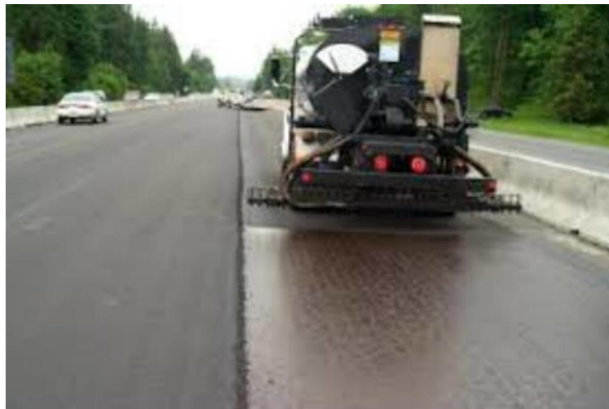
Figure 54. Photo of a Good Tack Coat (Courtesy of RoadResource.com)
