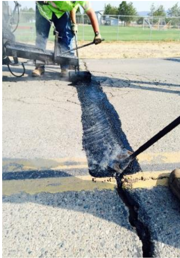
Figure 25. Mastic Placed in a Wider Crack (Courtesy of Maxwell Products)
