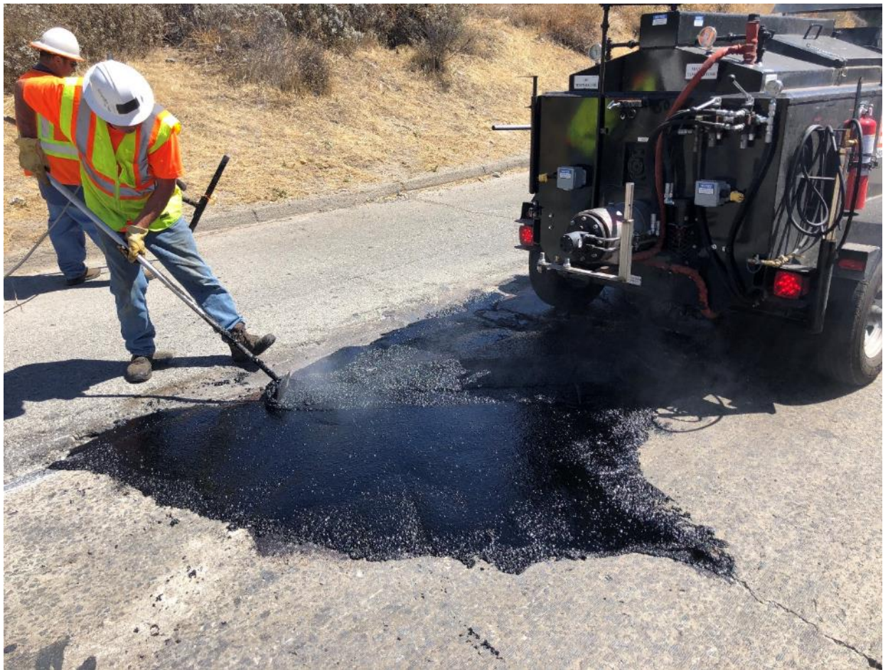
Figure 43. Hot Mastic Patching (Courtesy of Maxwell)
