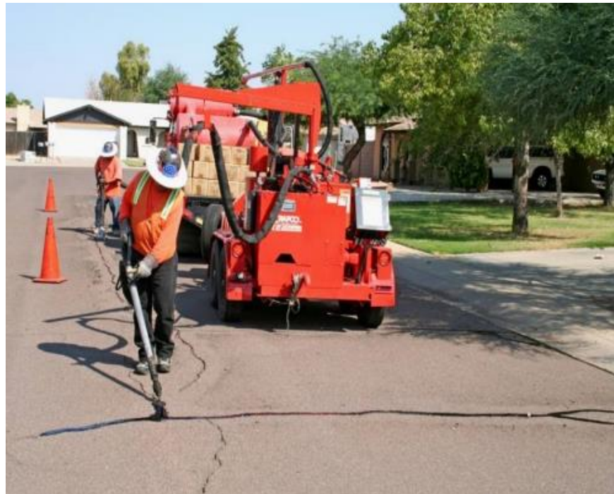
Figure 1. Common Crack Treatment (Courtesy of Crafc0)
