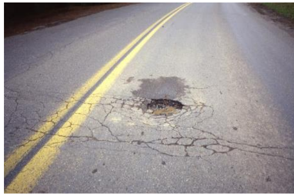
Figure 30. Typical Pothole
