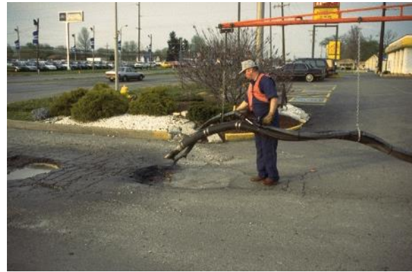
b) Application of Tack Coat
