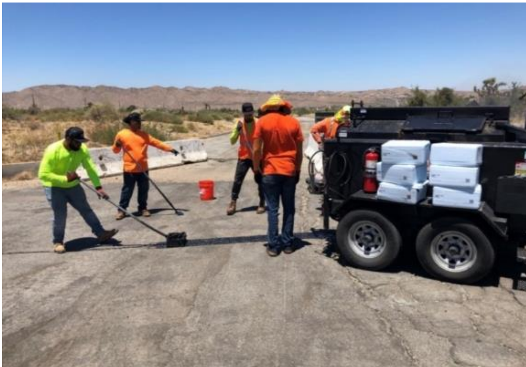
Figure 24. Application of Mastic in Wide Cracks (Courtesy of Maxwell Products)
