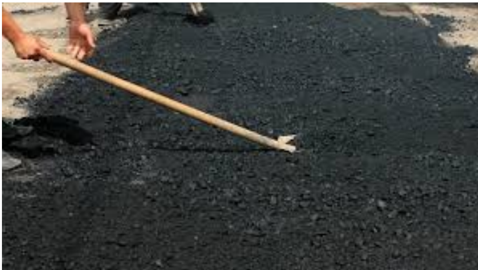
Figure 49. Hand Leveling of a Skin Patched Area
