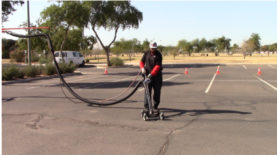
Figure 10. Vacuum Crack Cleaning (Courtesy of Crafc0)
