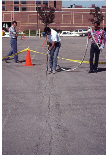
Figure 8. Air Blasting of Routed Crack (Courtesy of Crafc0)
