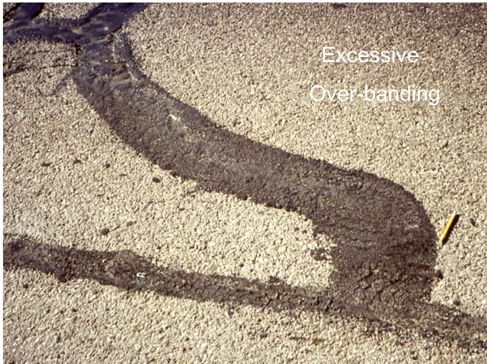
Figure 16. Excessive Overband
