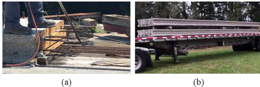
Figure 7.9: (a) Beam release stage and (b) delivery of slab-beam specimens
