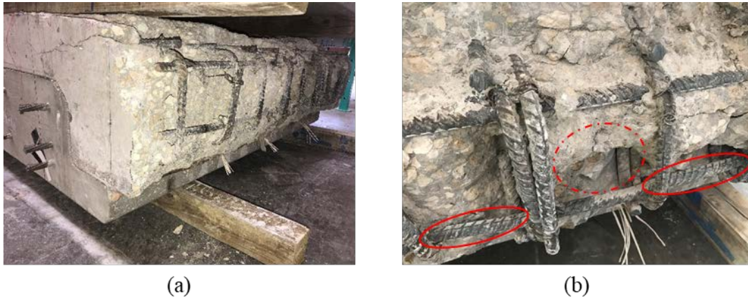
Figure 5.46: (a) Failed FSB Control-1 joint and (b) pull-out cavity in inner confined concrete (dashed line) and longitudinal rebar bend due to bending and pull-out forces (solid lines)
