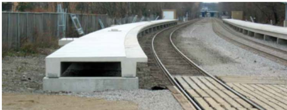
Figure 2.7: High-level railroad platform [7]
