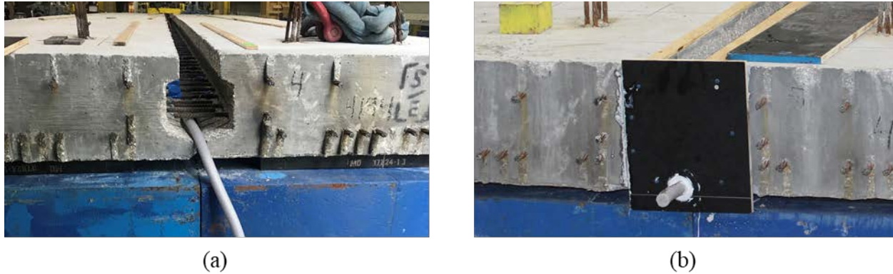
Figure 7.15: Backer rod detail: (a) 1-inch diameter rod and (b) rod extension through block-out form
