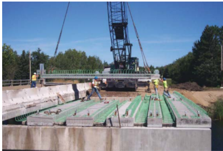
Figure 2.16: Erection of Bridge 04002 located on MN Highway 72 over the Tamarac River near the rural, northern Minnesota town of Waskish [11]
