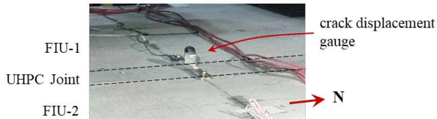
Figure 7.35: Crack displacement gauge used across joint
