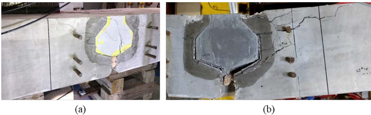
Figure 6.21: Failure crack for ultimate strength testing of 12A1 (a) without any fatigue load applied, 12A1-1 and (b) after fatigue loading, 12A1-2
