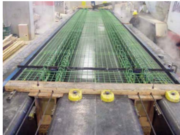
Figure 2.11: NEXT beam section at Dailey Precast plant, Shaftsbury, Vermont [7]
