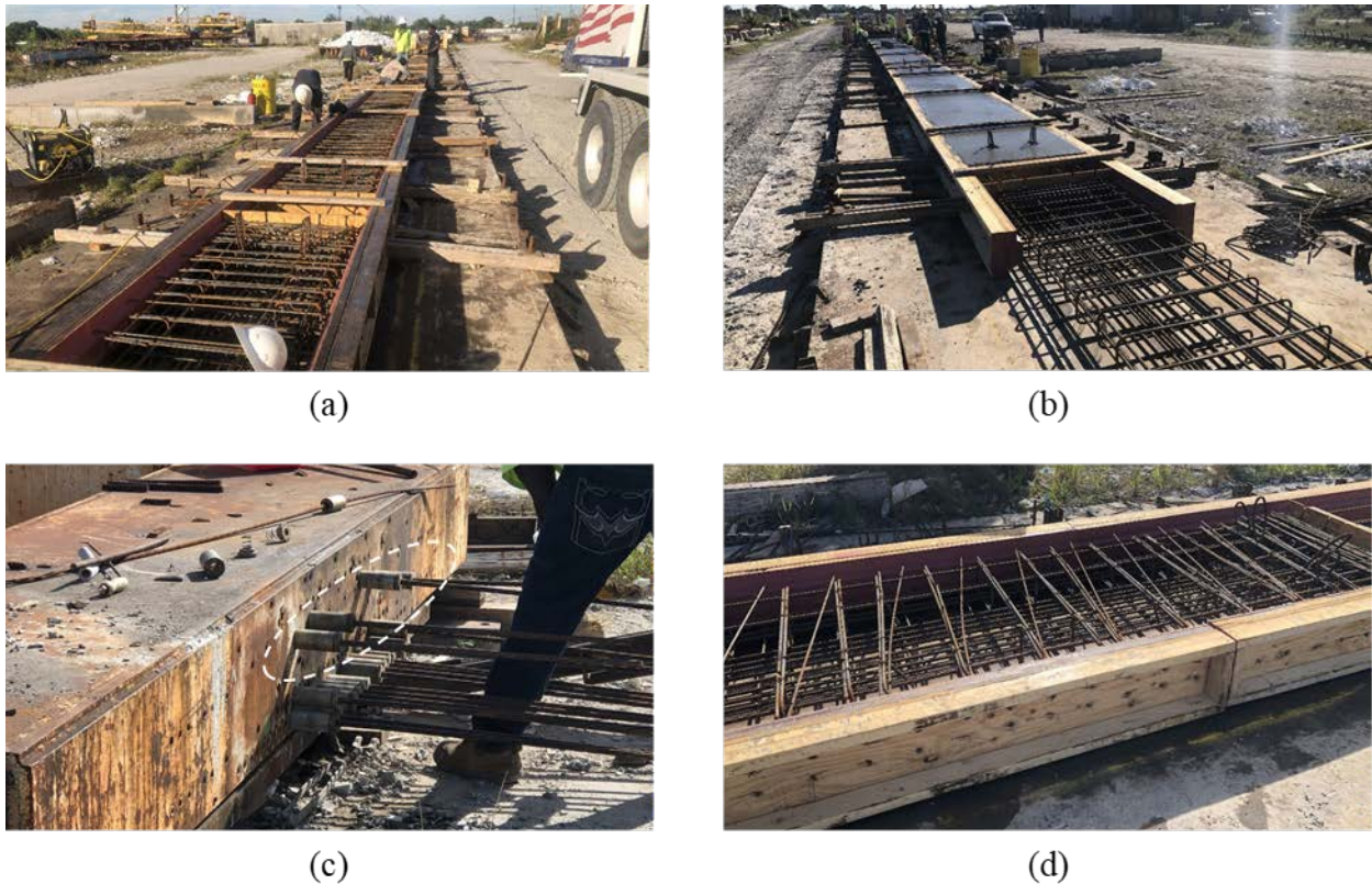
Figure 8.5: Construction of second set of beams: (a) FIU-8, FIU-7, and FIU-6 mild reinforcement and formwork construction, (b) concrete pour of first group of beams, (c) top strand layer de-tension, and (d) observed misalignment of mild reinforcement in second group of beams
