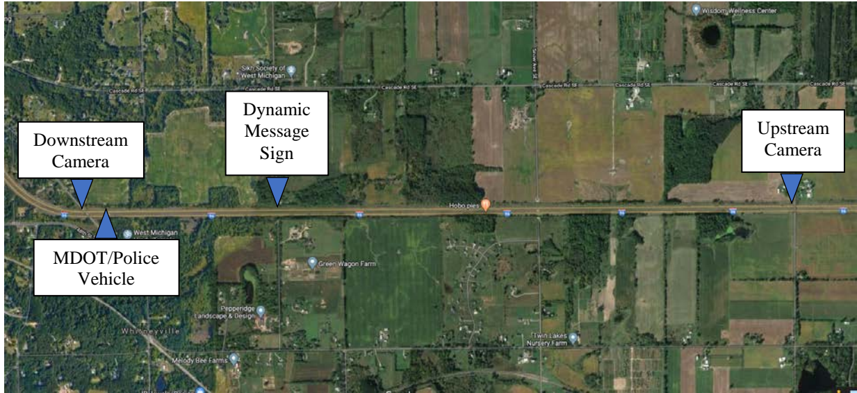
Figure 17. Westbound I-96 Highway Site
