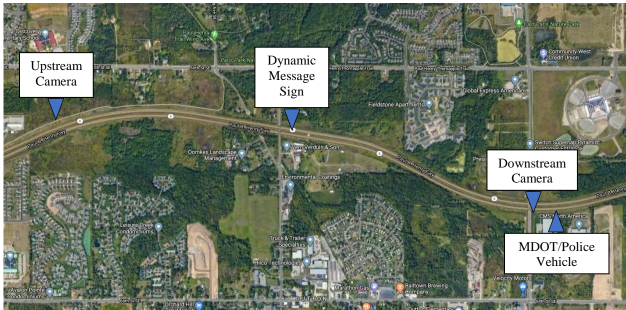
Figure 16. Eastbound M-6 Highway Site
