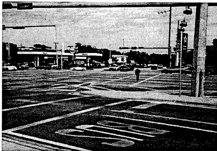
Figure 7.7 - "BUS ONLY" Pavement Marking at South Dade Busway At-grade Intersection
