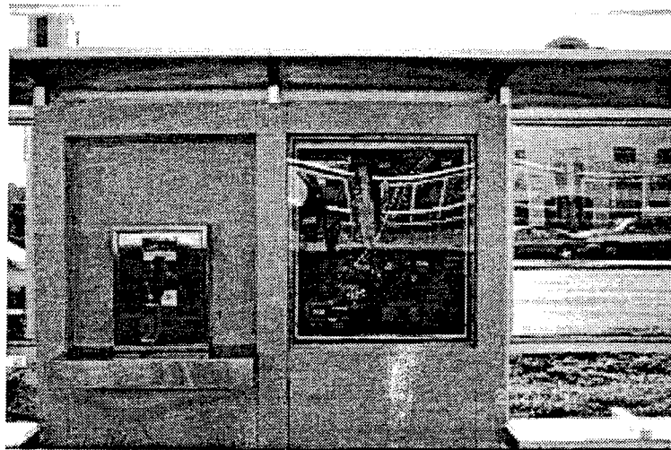
Figure 5.18 - Communication Facilities at South Dade Busway
