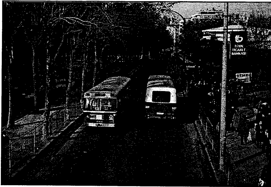
Figure 2.9 - Lateral Busway Using One Half of a Dual Roadway, Istanbul, Turkey Source: TRL, 1993
