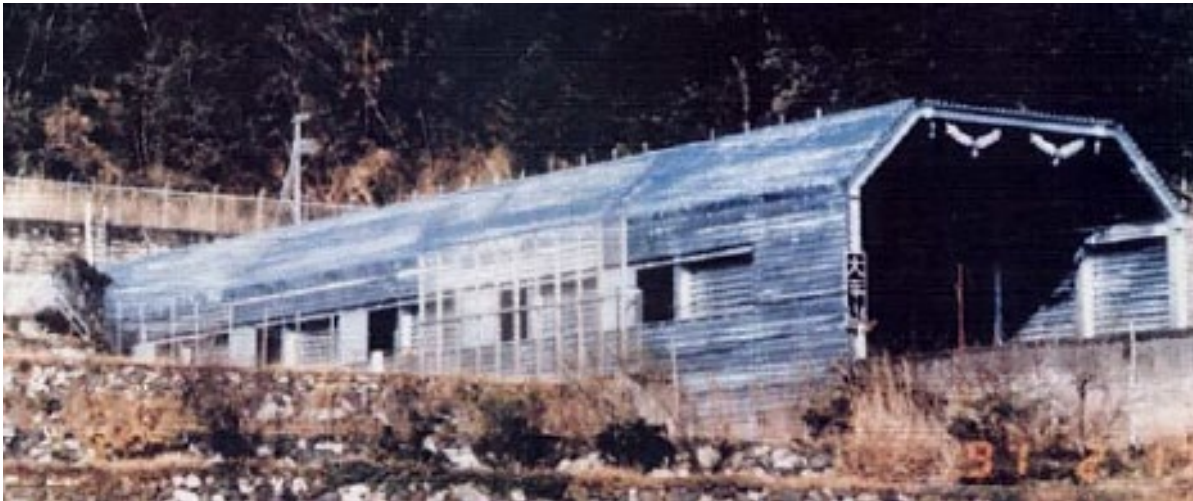
Figure 8-7. Japanese tunnel entrance hood (steel) – retro-fitted to Ohirayama tunnel, from Maeda et al [94]; reproduced by kind permission of the authors
