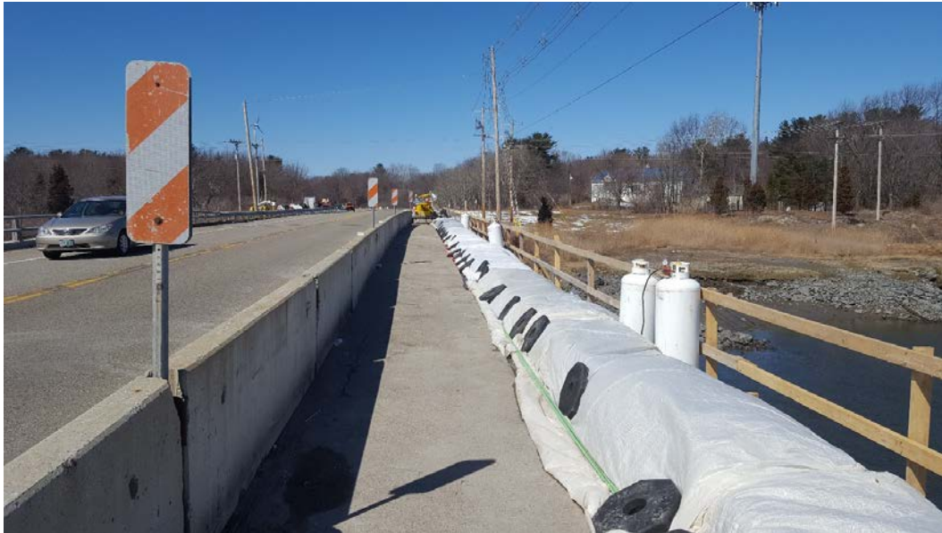
Figure 7: Insulated wrap and heaters on a bridge curb after cold weather placement.
