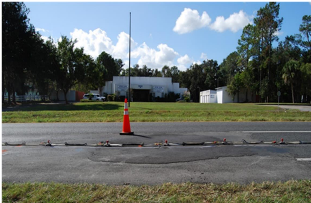
Figure 4.1. US-441 highway test site with a repaired sinkhole (pavement patched area)
