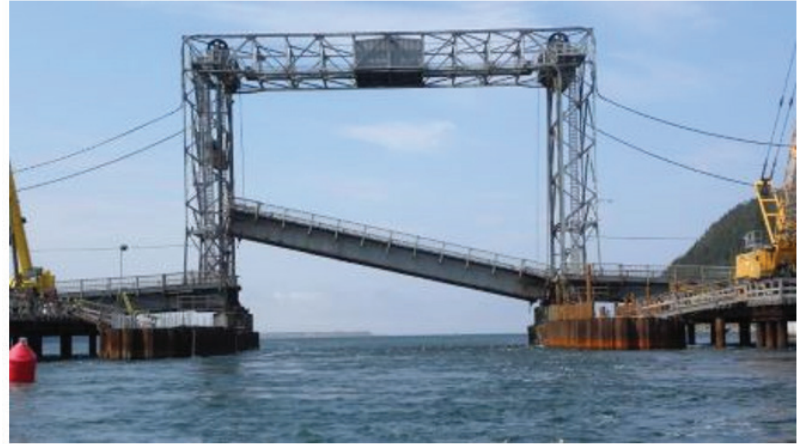
Figure 1. A vertical lift bridge rendered non-functional due to a severely skewed deck
