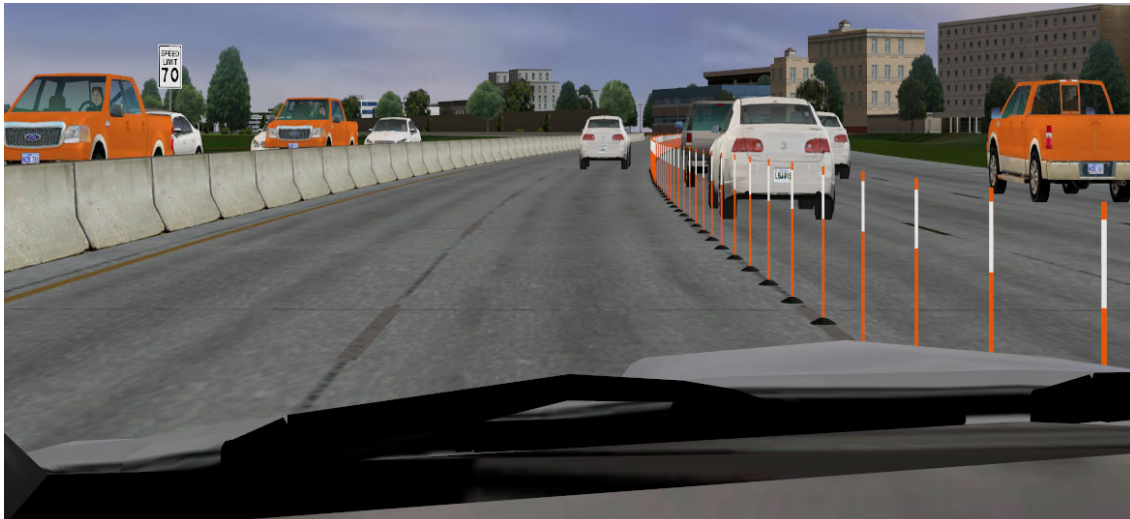
Figure 3-6: Orange Delineators with White Reflective Sheet and Concrete Surface
