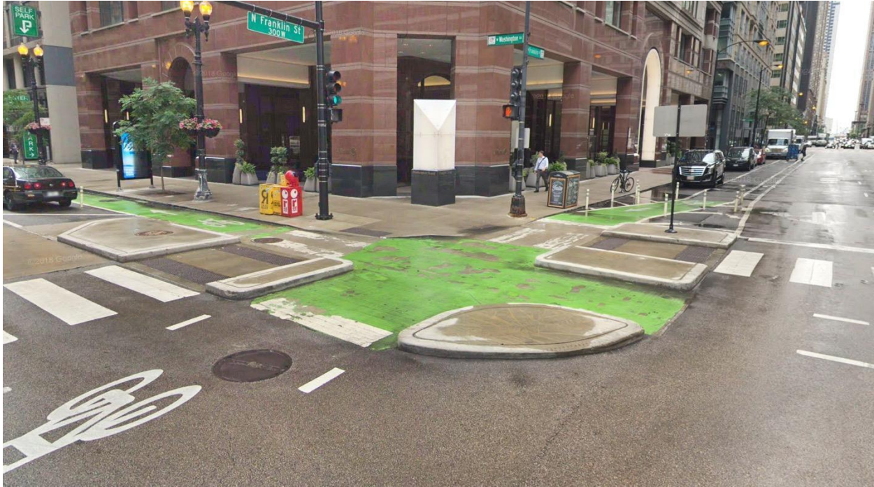
Figure 4.11 Chicago Protected Intersection (Source: Alta Planning + Design, 2015)
