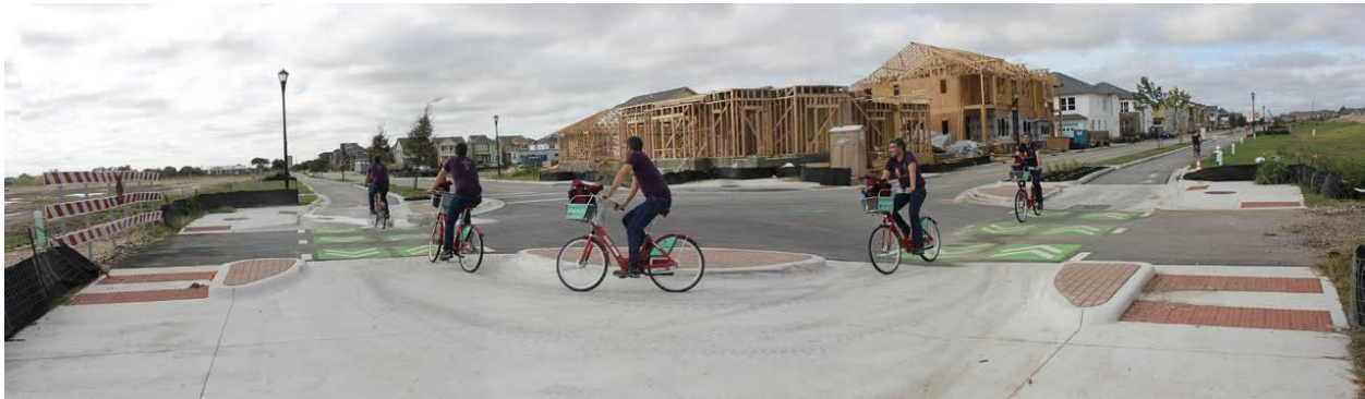
Figure 4.9 Austin Protected Intersection (Source: Alta Planning + Design, 2015)
