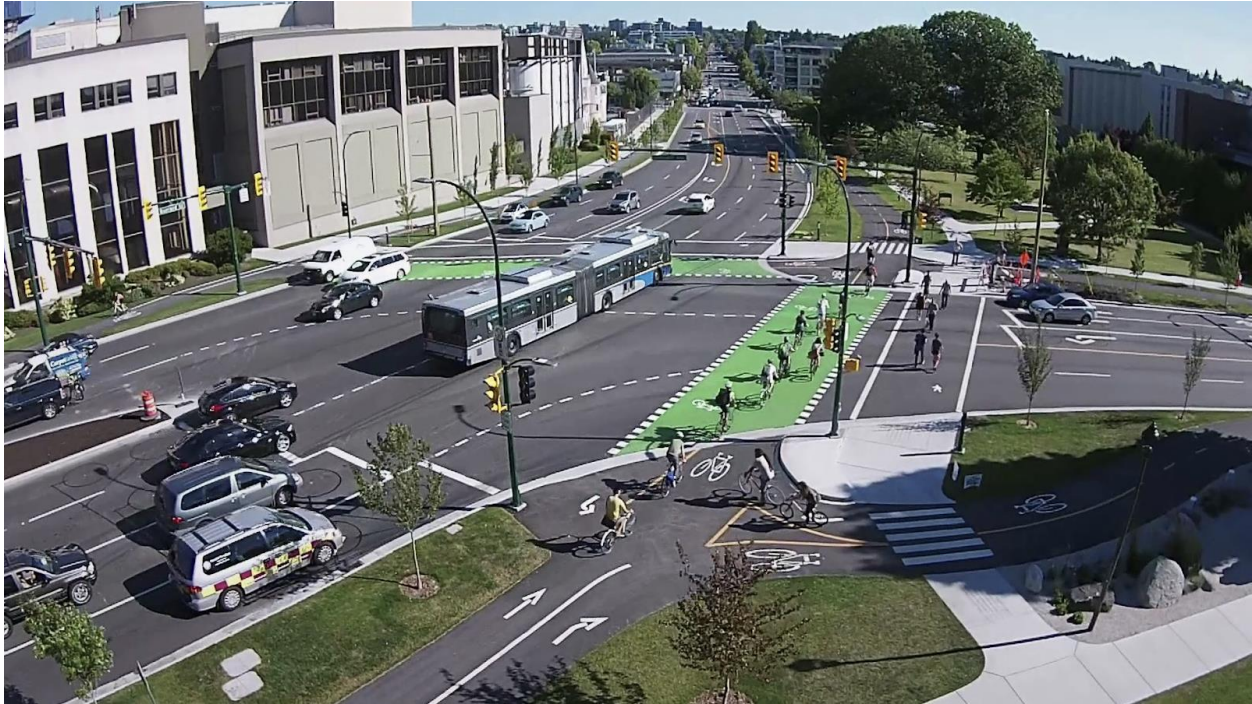
Figure 4.12 Vancouver Protected Intersection (Source: Alta Planning + Design, 2015)
