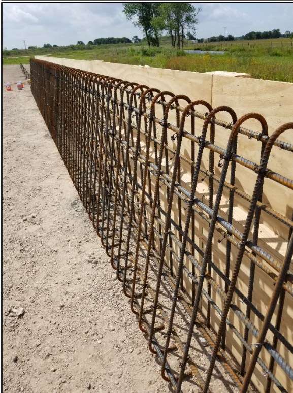
Figure 3.2. SSCB with the Drilled Shaft Foundation Construction.
