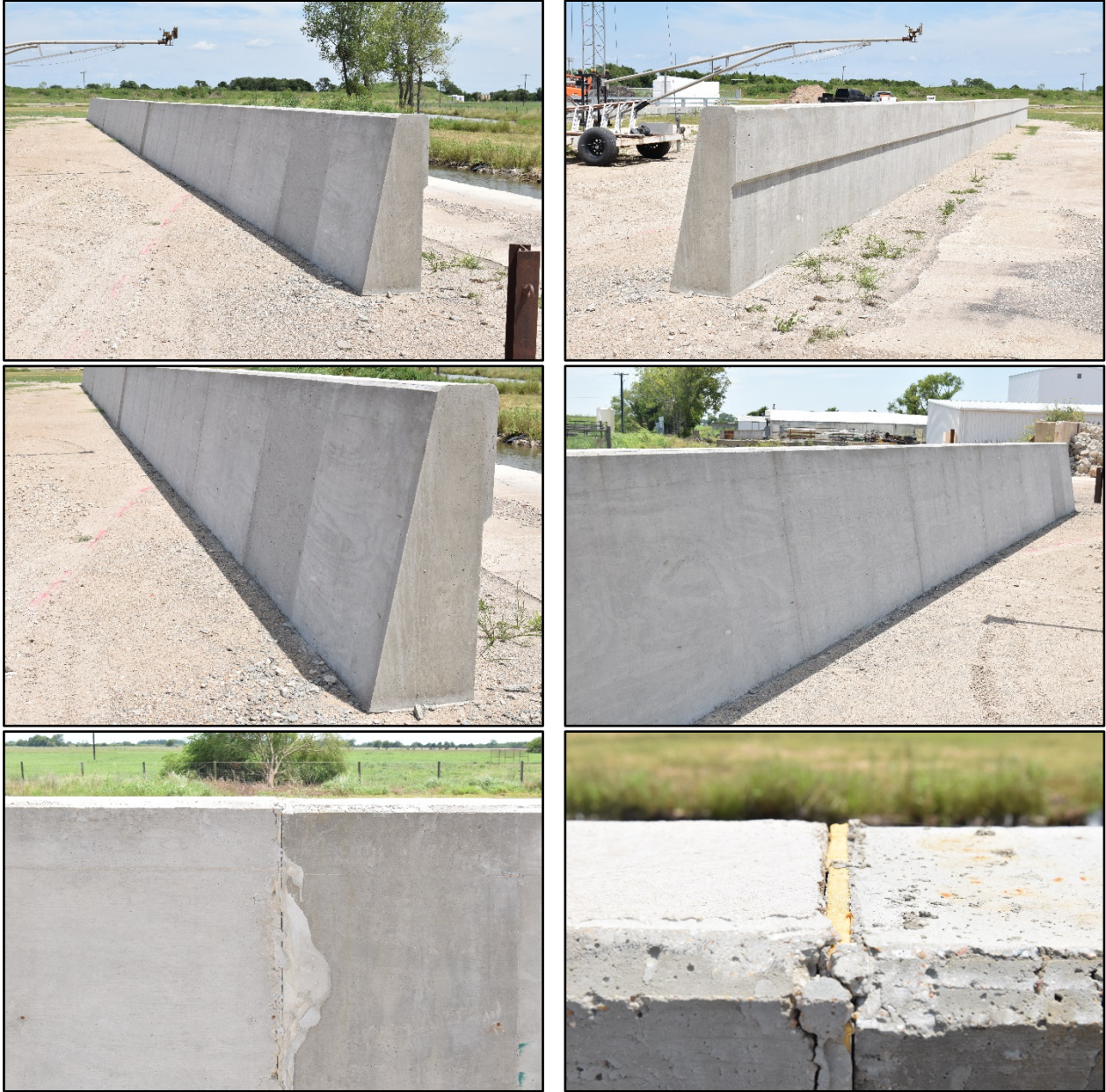
Figure 3.3. SSCB with the Drilled Shaft Foundation prior to Testing.
