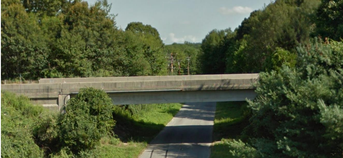
Figure 2.4: South elevation of the Lebanon Bridge, CT-2 Westbound (Google Maps, 2017)
