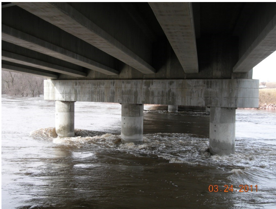
Figure 7.4 Bridge crossing from right bank facing bent 2 of southbound bridge
