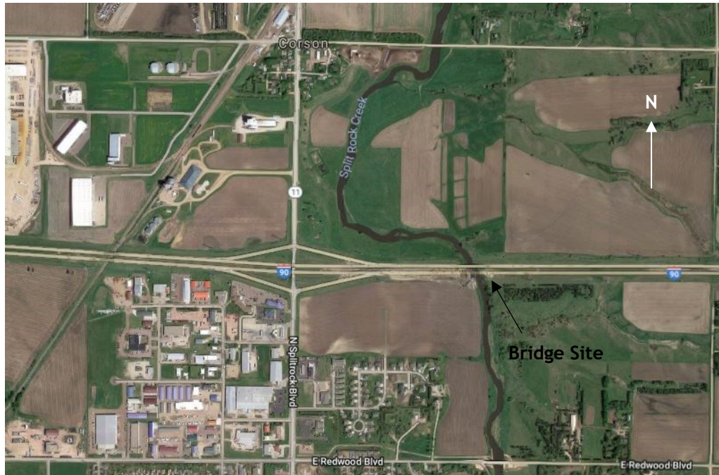
Figure 8.1 Aerial photograph of Interstate 90 bridges over the Split Rock Creek near Brandon, South Dakota
