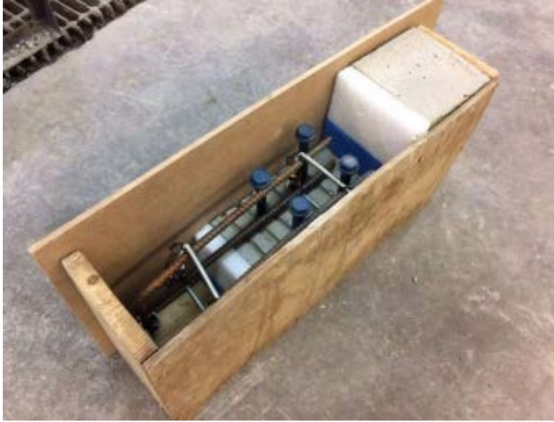
Figure 13: Underlay half with anchors protruding from the bond surface prior to pouring of overlay concrete
