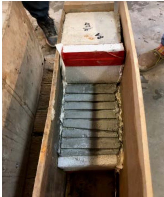
Figure 11: Underlay half with bonding agent applied on the bond interface just before pouring of overlay concrete
