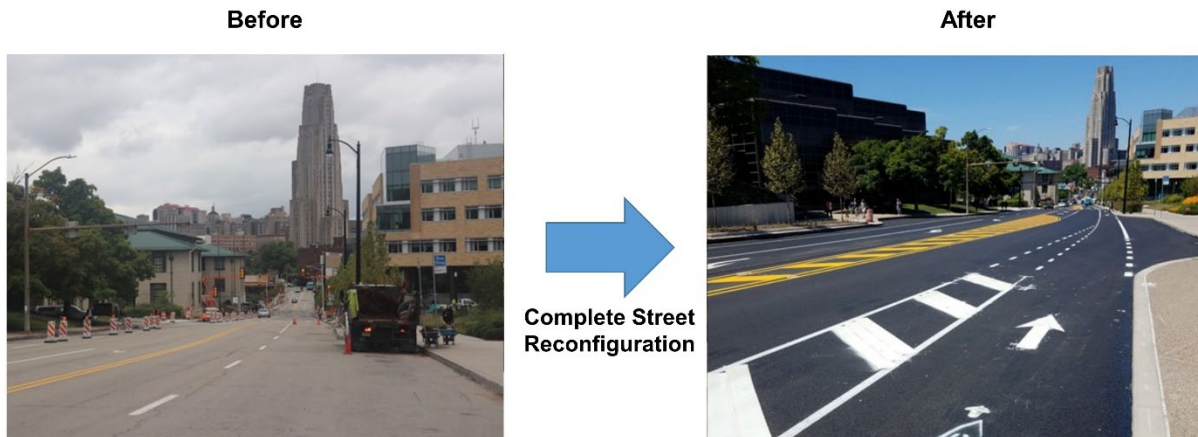
Figure 2 - Pre- and post-retrofit images
