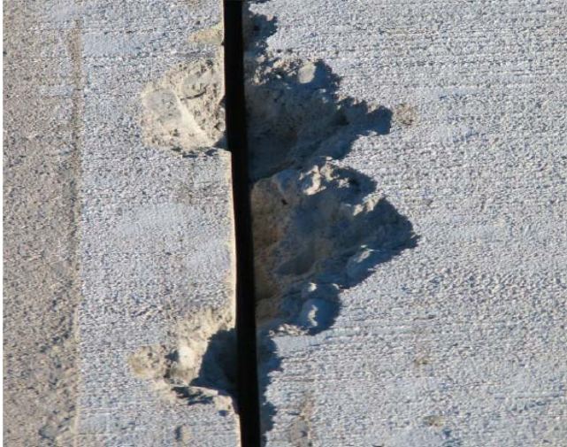
Figure 1.2.5. Raveling due to Poor Sawing Practice (Source: Iowa Department of Transportation)
