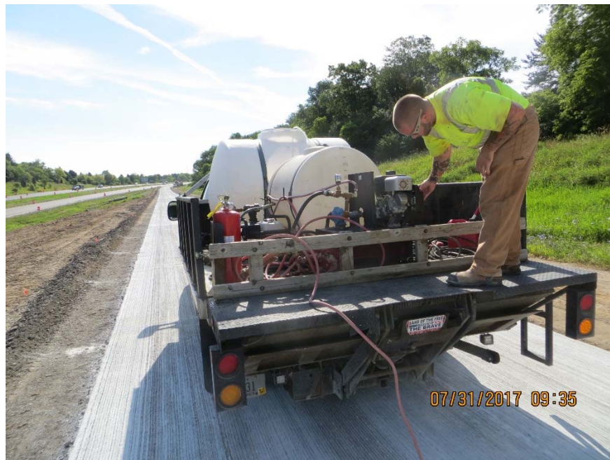
Figure 2.10.15. Truck-Mounted Joint Sealing Equipment
