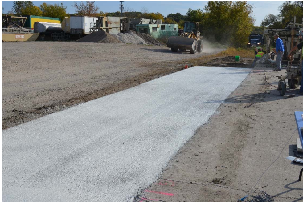
Figure 2.5.6. Application of Curing Compound Over Gravel Mixture
