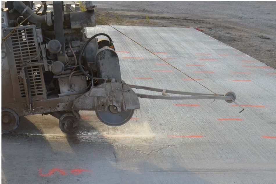
Figure 2.5.17. Initial Conventional Saw Cut in Limestone Mixture (Joint 11)
