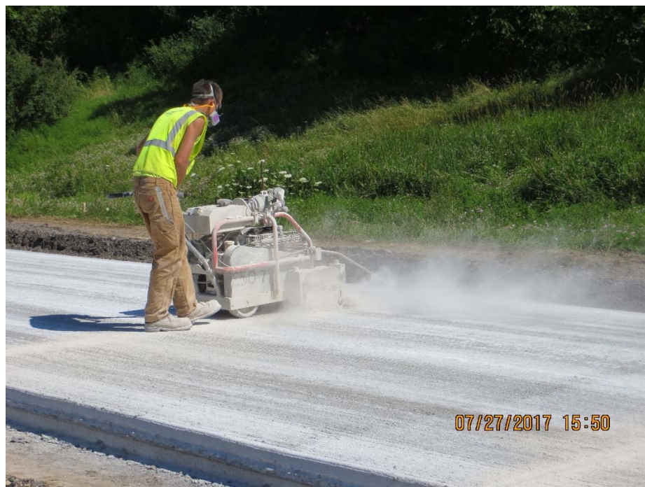
Figure 2.10.14. Husqvarna SOFF-CUT Model 4000 Early Entry Sawing Operations
