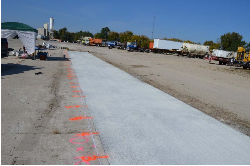
Figure 2.5.7. Overview of Completed Test Sections with Joint Location Markings
