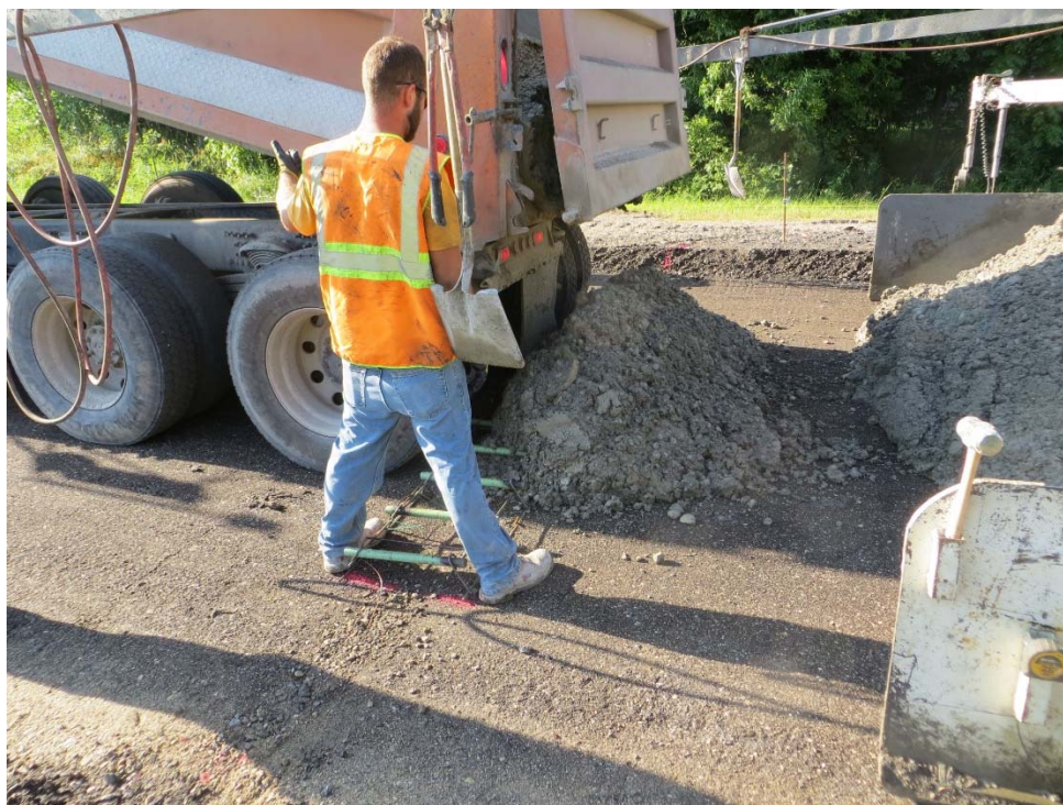
Figure 2.10.4. Placement of Concrete Over Dowel Basket
