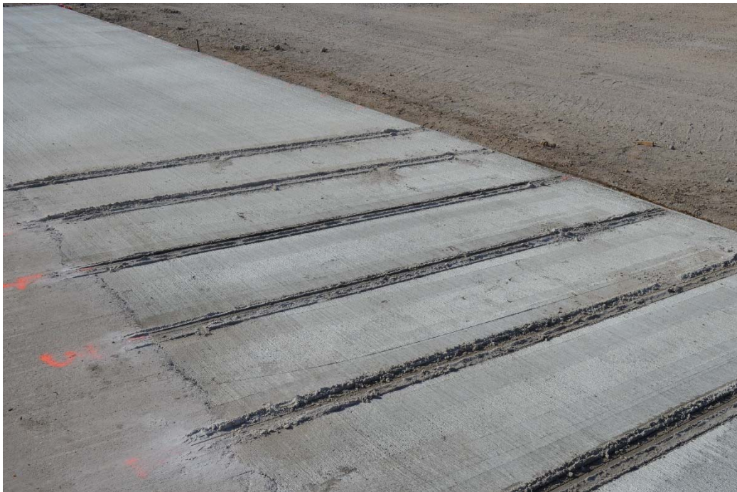
Figure 2.5.16. First Six Early Entry Saw Cuts in Limestone Mixture
