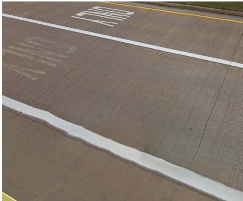
Figure 5.4.1. Well Performing Joint Conditions Along CTH OO-P1, East of STH 124, November 2015
