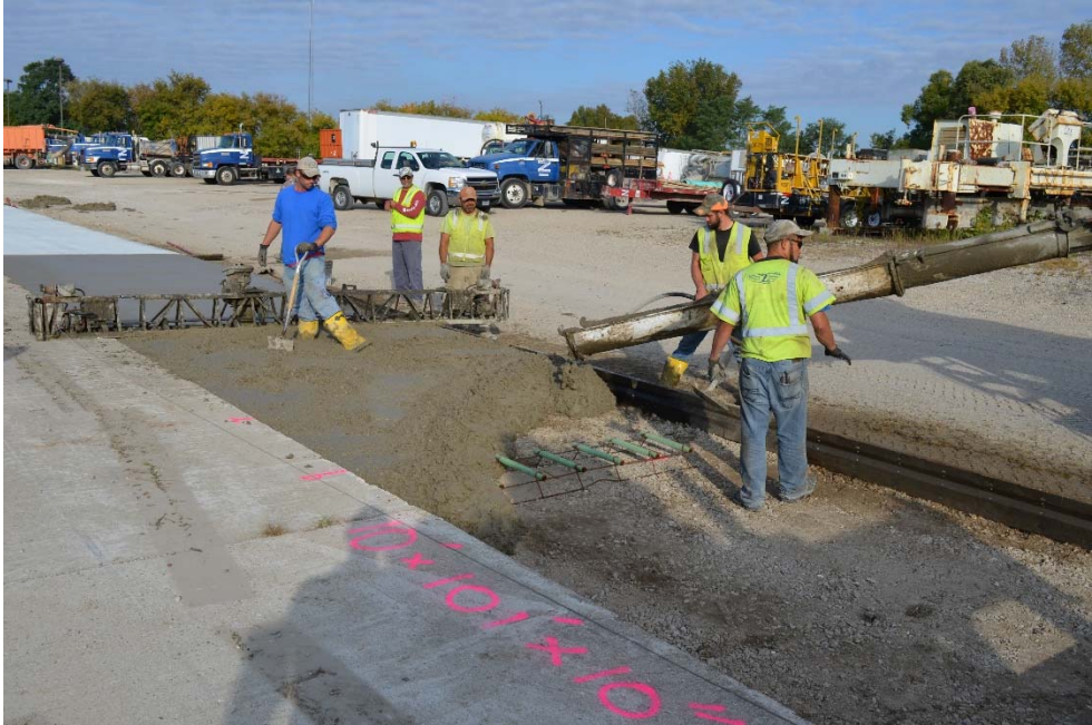
Figure 2.5.5. Paving Operations Within Gravel Mixture Near Dowel Basket
