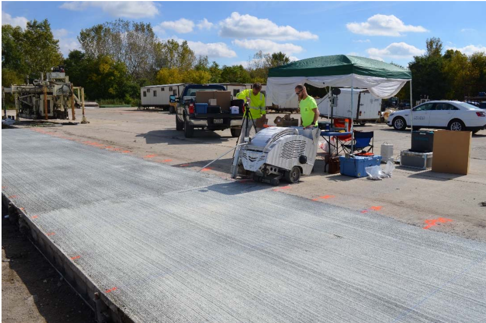
Figure 2.5.8. Preparations for Initial Saw Cutting in Limestone Mixture
