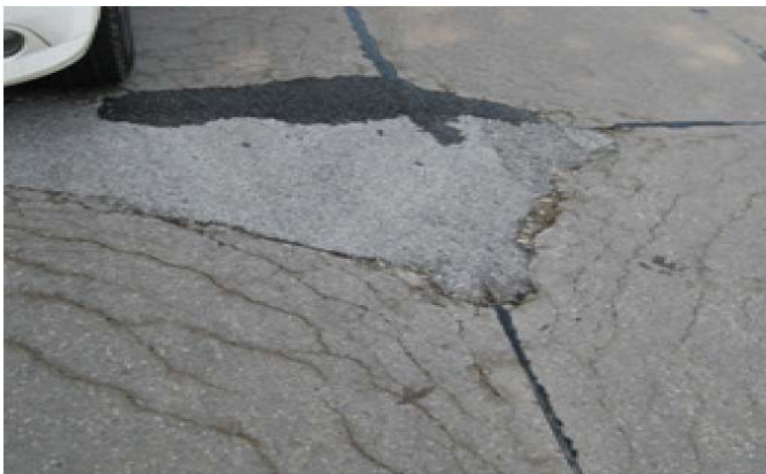
Figure 1.2.6. D Cracking of High Severity (Source: The Transtec Group)
