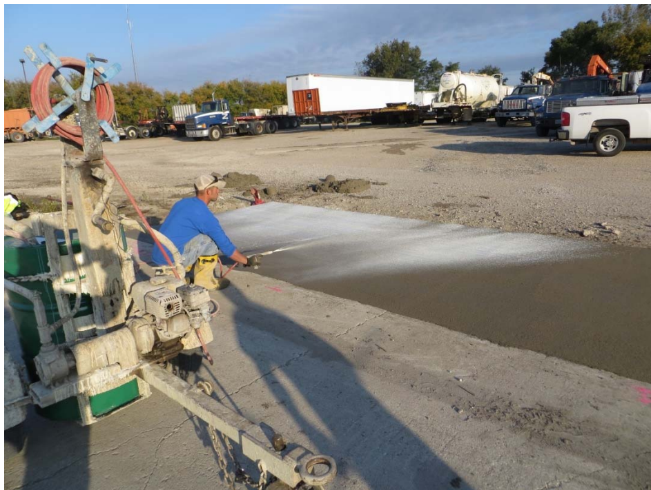
Figure 2.5.4. Application of Curing Compound Over Limestone Mixture
