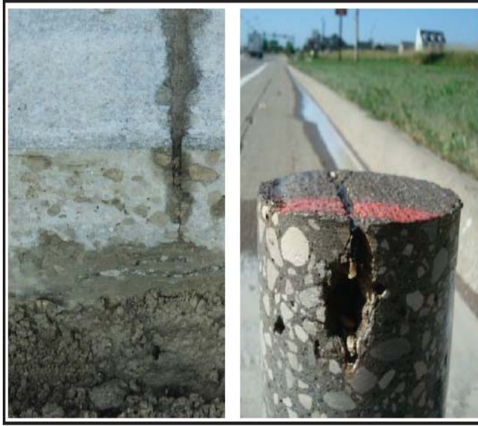
Figure 1.2.2. Saturated Soils due to Inadequate Drainage and Roadside Irrigation (left) Leading to Joints Showing Frost Damage (right) (Source: Snyder and Associates)
