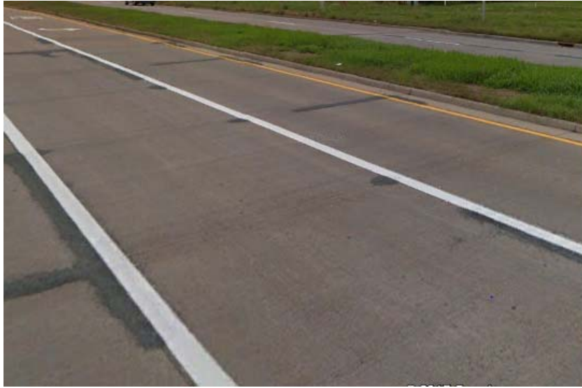
Figure 5.4.1. Deteriorated Joint Condition Along CTH OO-P2, Just East of STH 124, November 2015
