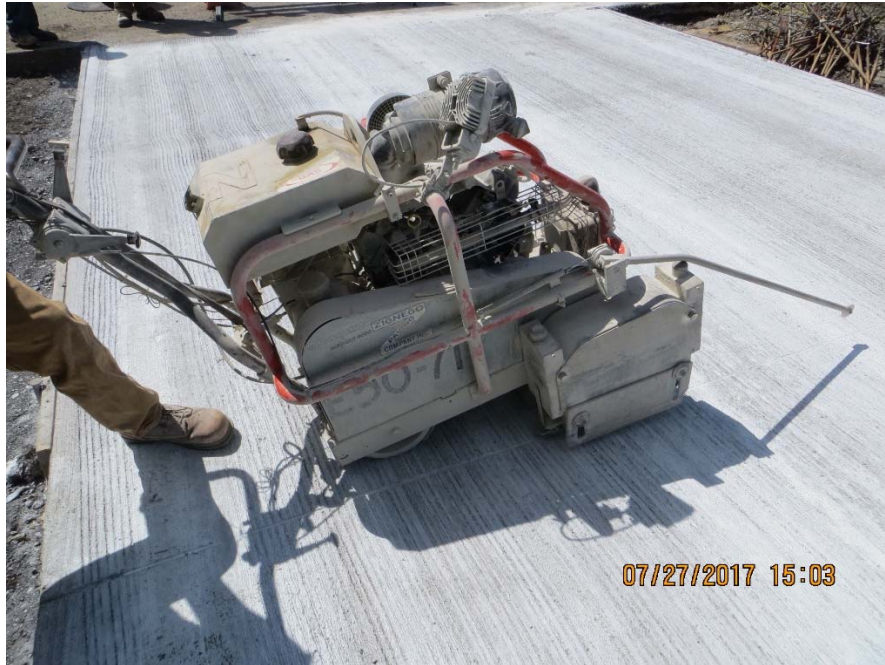
Figure 2.10.13. Husqvarna SOFF-CUT Model 4000 Early Entry Saw
