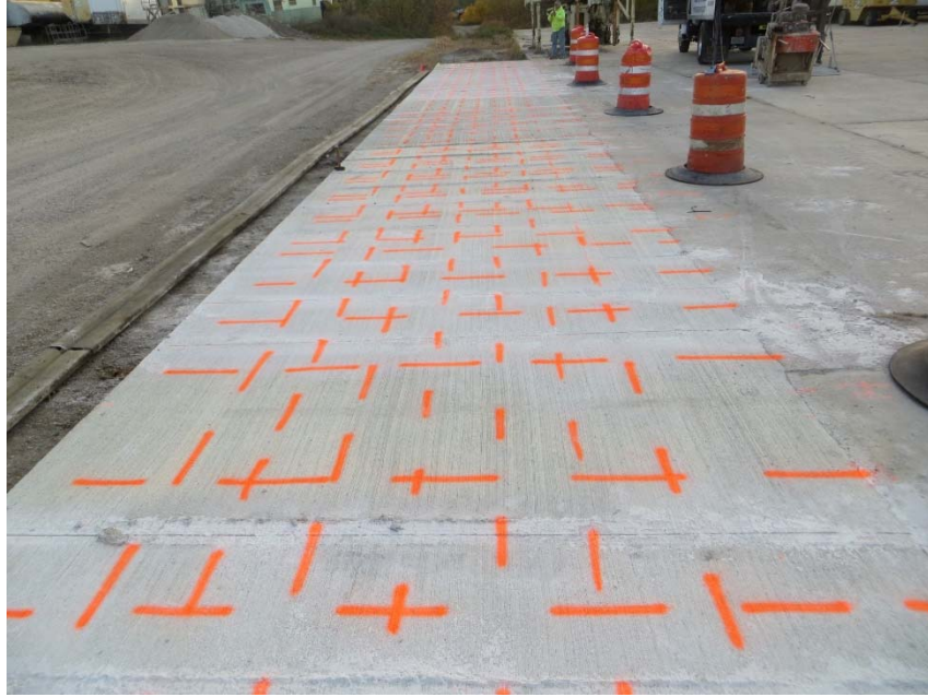
Figure 2.6.2. Layout Markings For Full-Depth Sawing
