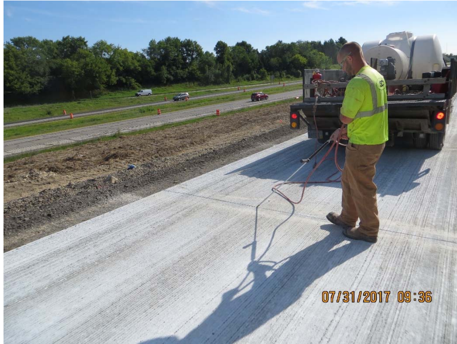
Figure 2.10.16. Joint Sealing Operations
