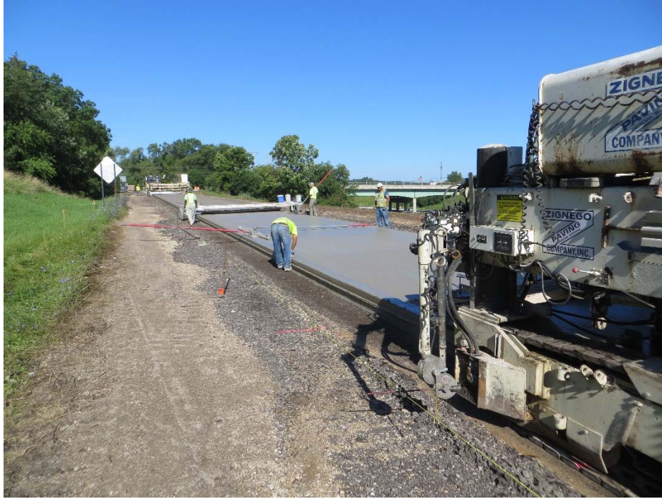
Figure 2.10.5. Complete Paving Train with Paver, Turf Drag and Tiner/Curing Compound
