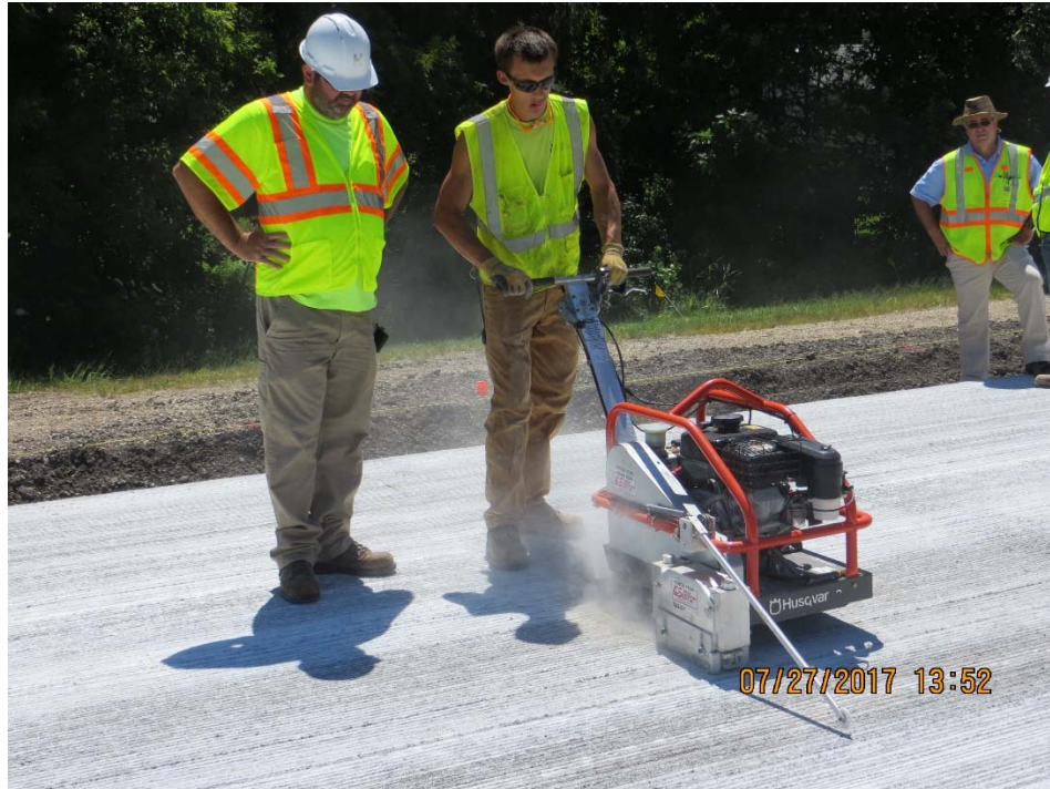
Figure 2.10.12. Husqvarna SOFF-CUT Model 2000 Early Entry Sawing Operations
