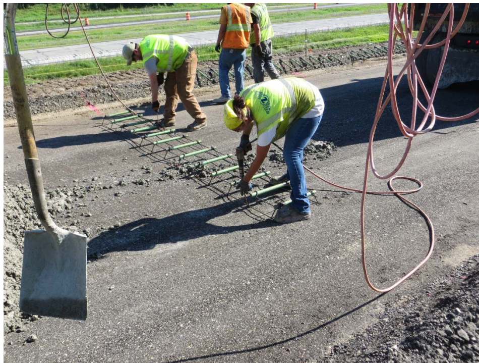
Figure 2.10.3. Placement of a Dowel Basket in Advance of Mix Placement
