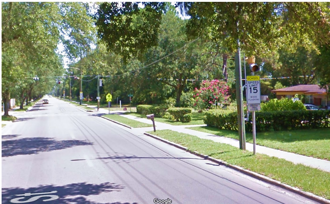
Figure 1 Intelligent school beacon on NE 15th St. controlled by the AI/Glance system (Beacon 4.1 in this study)
