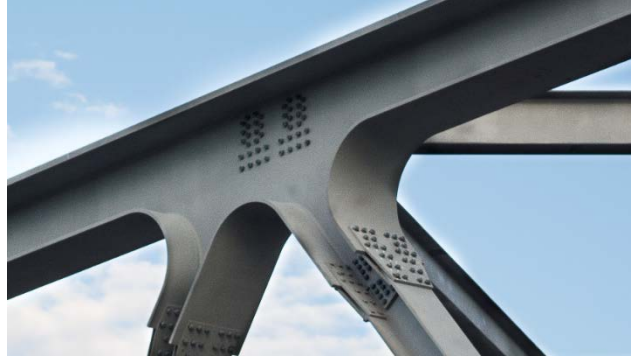
Figure 8. The gusset-less connection at the Memorial Bridge connecting Portsmouth, NH and Kittery, ME.
