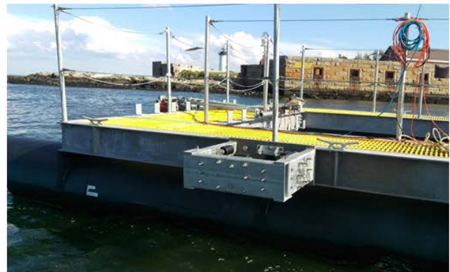
Figure 55. Pile guide mooring system.
