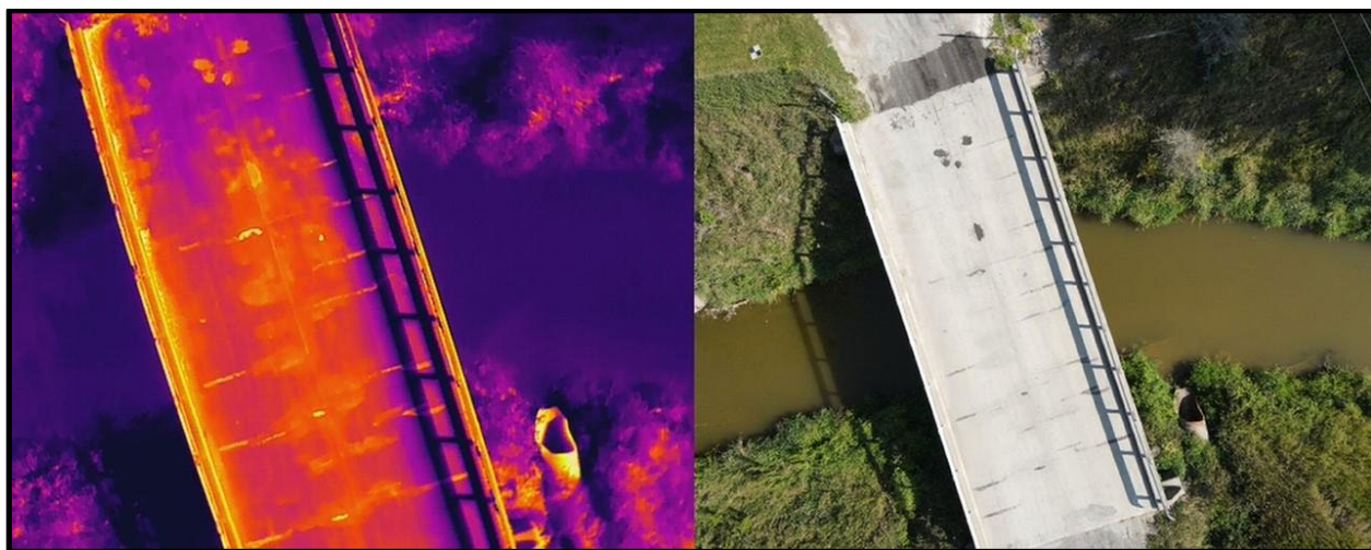
Figure 3.2.1: Beyer Road bridge, near Saginaw, MI, showing thermal data (left) and optical data (right) from the August 17, 2021 data collection.
