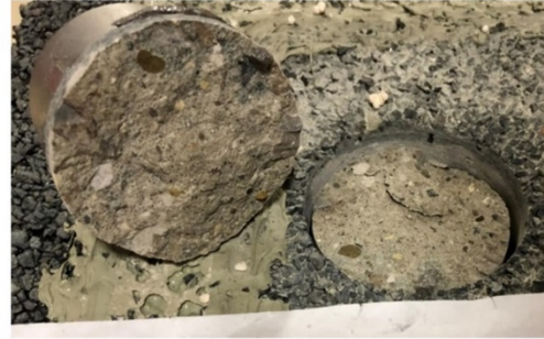
ii) Failure at room temperature following a wet cycle
