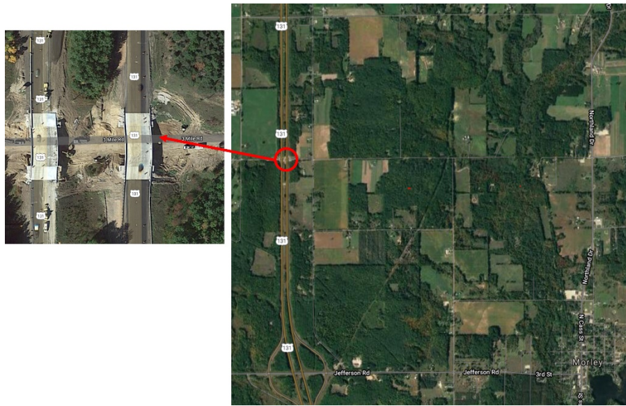
Figure 5-3. US-131 over 3 Mile Road bridge (43.511442, -85.485965) (Google map)
