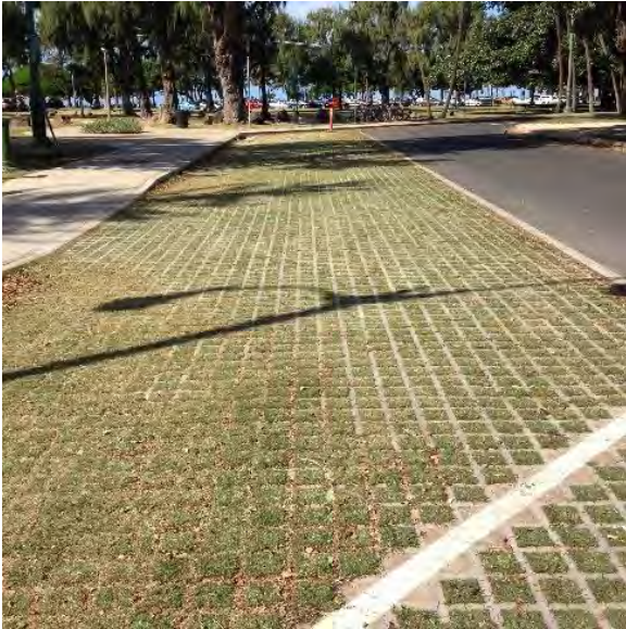
Figure 68 Permeable grass-crete in parking lot in Honolulu, HI. Photo: W. Meguro
