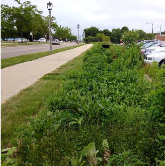
Figure 52 Bioswale between the roadway, sidewalk, and parking lot in Milwaukee, WI. Photo: W. Meguro
