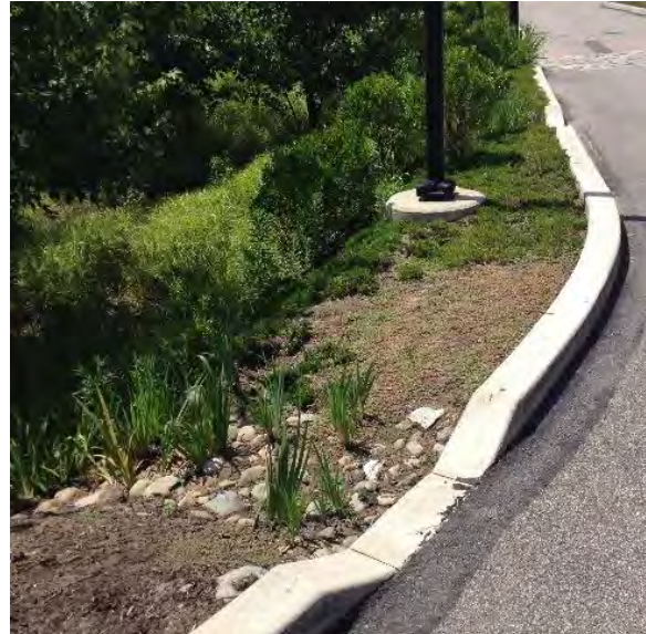
Figure 55 Bioswale, curb, cut, and pervious asphalt at the Center for Sustainable Landscapes in Pittsburgh, PA. Photo: W. Meguro
