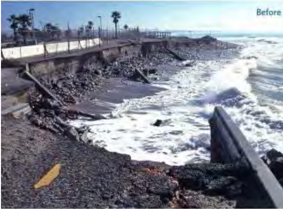
Figure 16 Site in California before landward realignment of built infrastructure and restoration of the dunes and beach. The bike path and parking lot were built on fill in 1989 and eroded within 2 years. Source: Judge, J. et. al. xxxv
