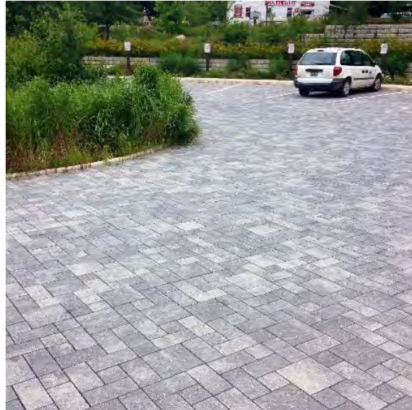
Figure 69 Permeable paving in parking lot in Pennsylvania. Photo credit: W. Meguro
