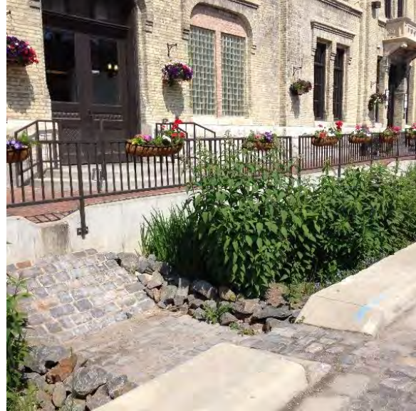
Figure 53 Bioswale with curb cuts adjacent to urban buildings, sidewalk, and road in Milwaukee, WI. Photo: W. Meguro
