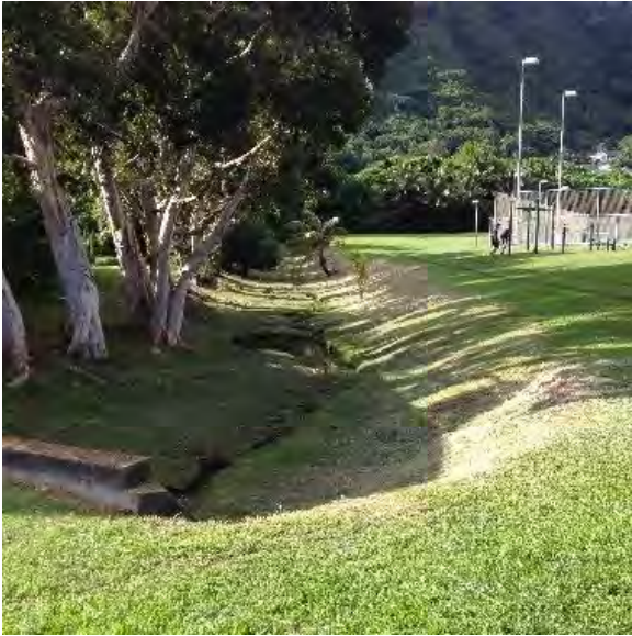
Figure 60 Green space with swale in Honolulu, HI. Photo: W. Meguro.
