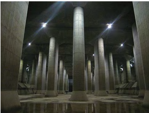
Figure 70 Water storage tank in Japan's G-Cans project. Source: Dddec0.
