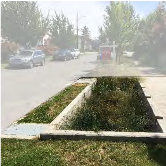
Figure 54 Vegetated stormwater detention basin in Seattle, WA. Photo: W. Meguro
