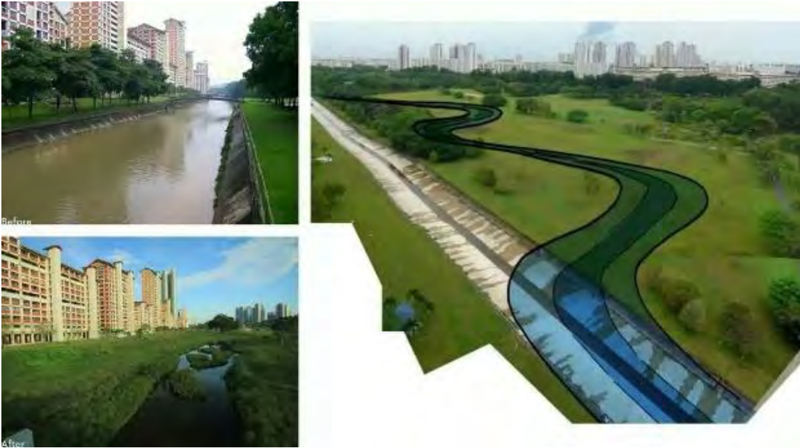
Figure 64 A stream de-channelization and park project in Singapore is a useful precedent for Wailani Stream and Kapakahi Stream in Waipahu.
