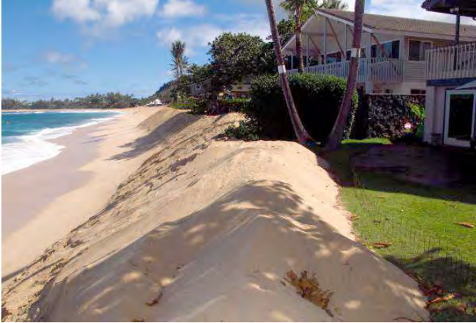
Figure 14 Newly restored dunes on O'ahu's North Shore protected homes from high waves during the 2015–2016 winter. xxxiii Source: Hawai'i Sea Grant.
