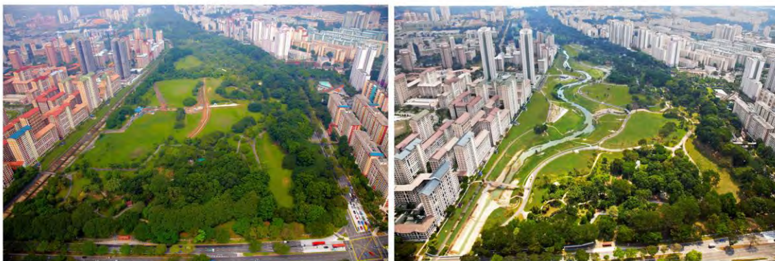
Figure 65 Before and After Kallang River de-channelization. xc
