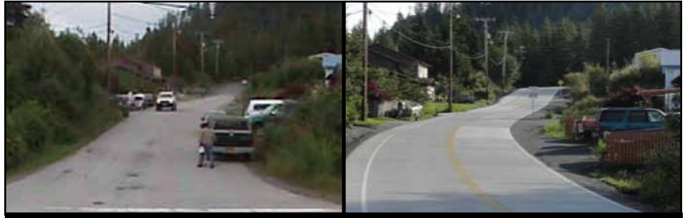
Prior to the Shtax-Heen Roadway Project, the associated roadways did not include accommodations for pedestrians. (Courtesy of the WCA) The Shtax-Heen Roadway Project includes paved roadways and pedestrian walkways (Courtesy of the WCA)
