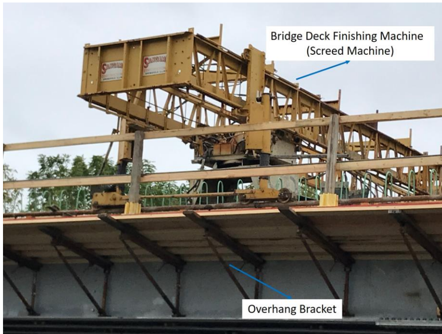
Figure 1. Construction of deck overhang.
