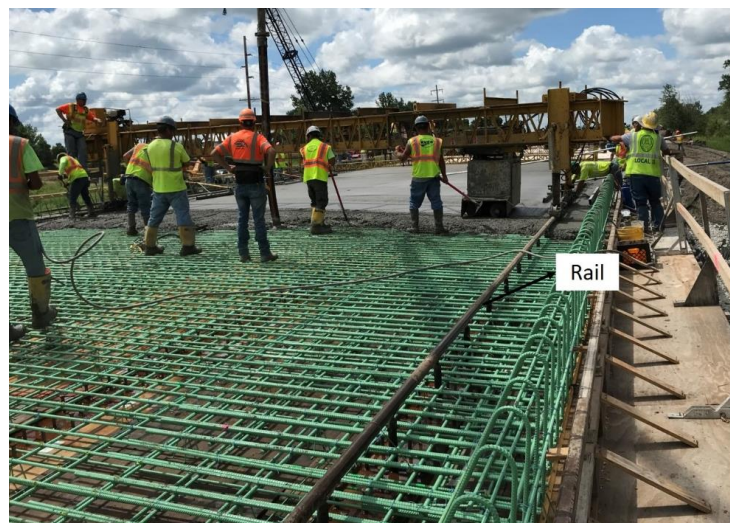
Figure 8. Screed-machine rail located at the center of exterior girder.
