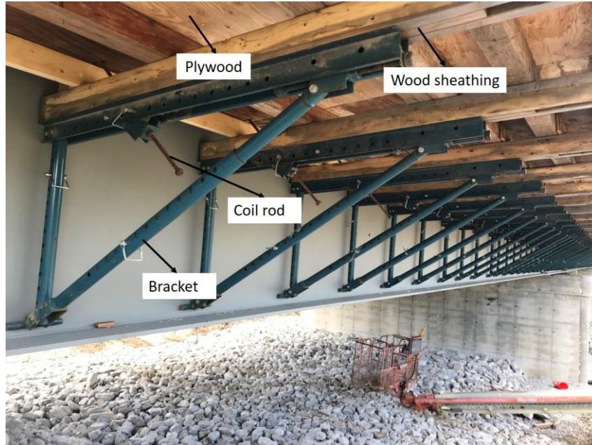
Figure 5. Overhang formwork.
