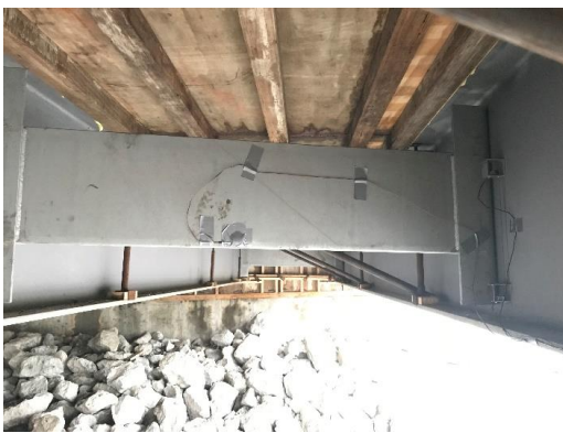
(c) Diaphragm with partial-depth connecting plate
