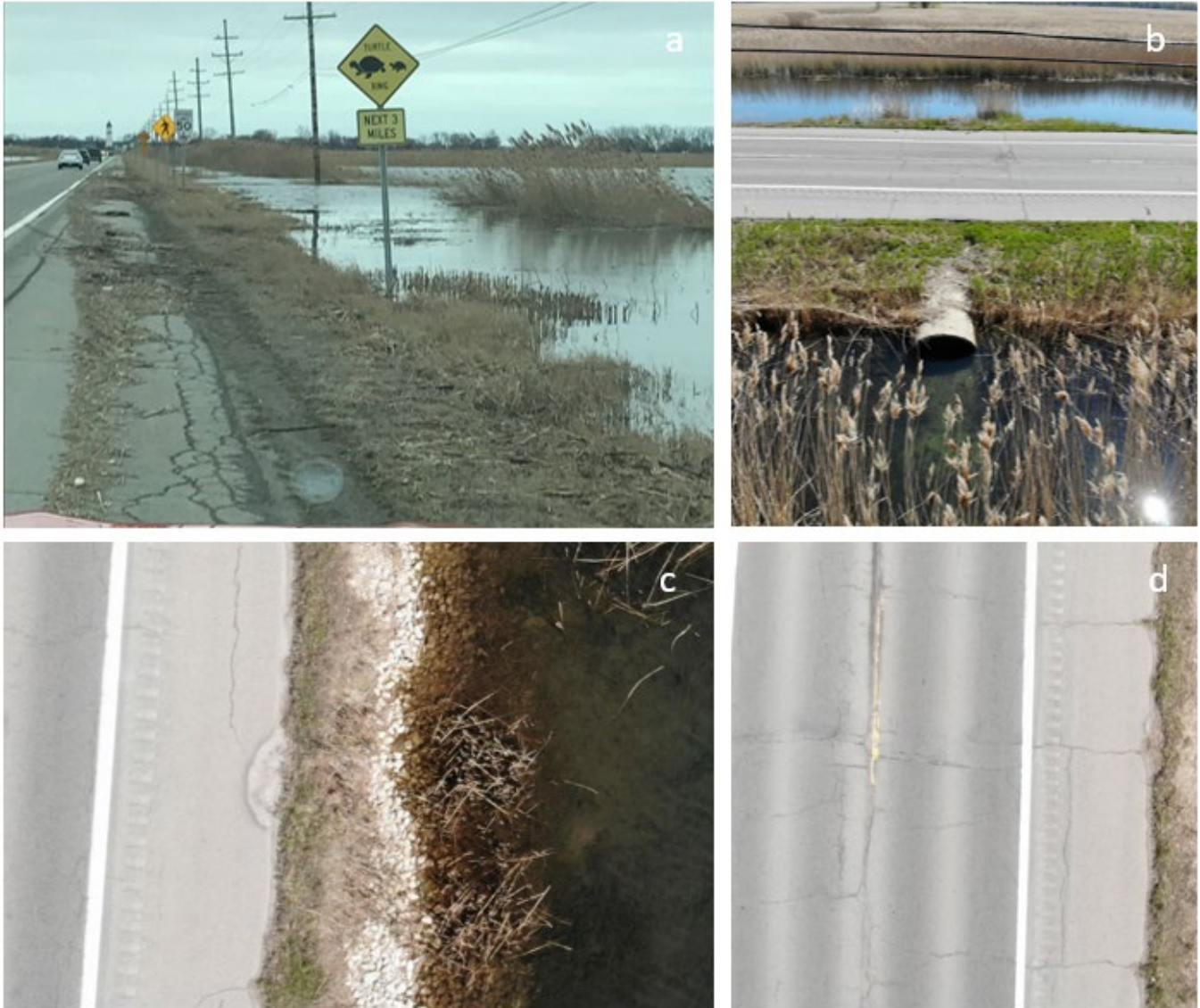
Figure 4-7. Historic flooding and current condition of roadway. a) debris showing extent of high water that has since receded (as well as an unapproved “turtle crossing” sign), b) a pipe culvert, one of the two culverts along the 5,800 feet considered, c) evidence of muskrat damage on the shoulder, d) typical cracking and rutting of this section of roadway.
